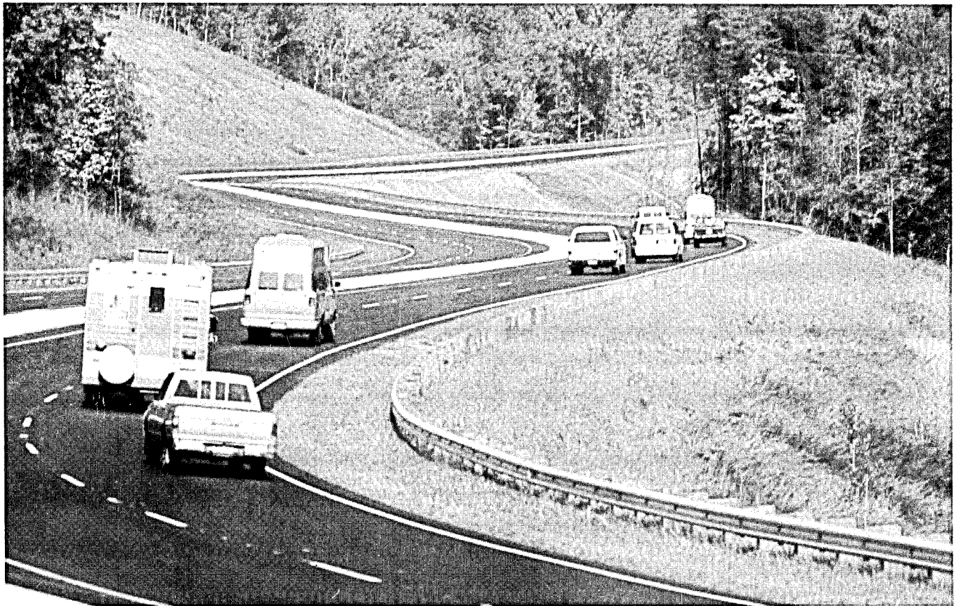
This four-lane section of US-221 and NC-226 in McDowell County near Marion opened to traffic on October 16, 1990.
