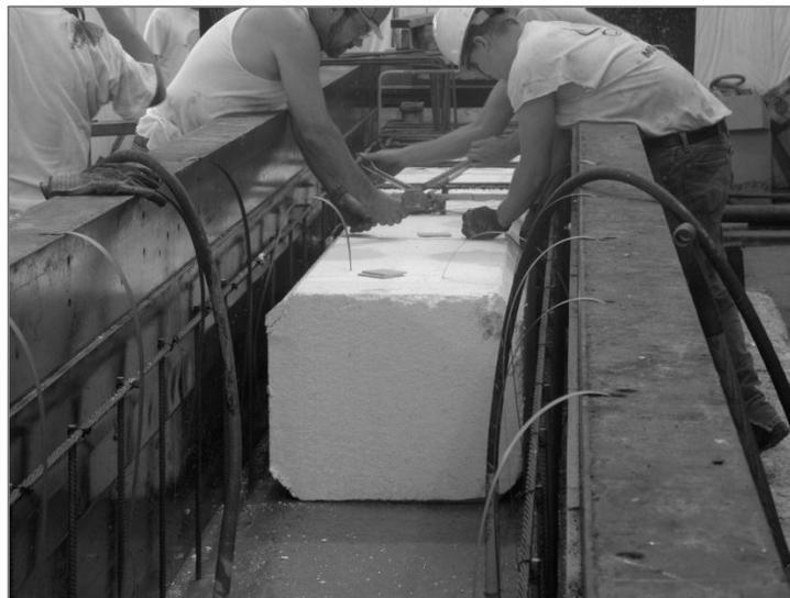
**Figure 5-7** Expanded polystyrene void forms are placed in the casting bed during casting of box beams.
