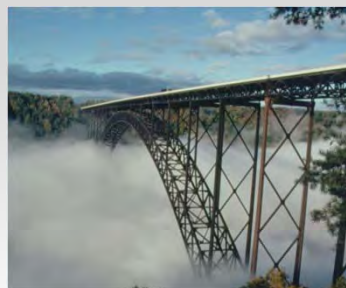
New River Gorge Bridge, WV (1700 ft main span)
