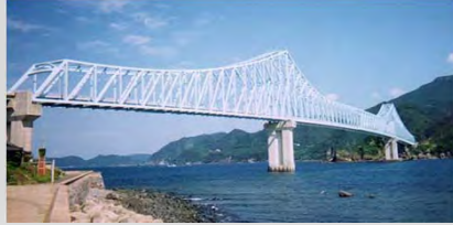
Ikitsuki Ohashi Bridge, Nagasaki, Japan (1300 ft main span)
