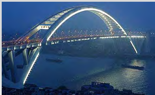
Lupu Bridge, Shanghai, China (1800 ft main span)
