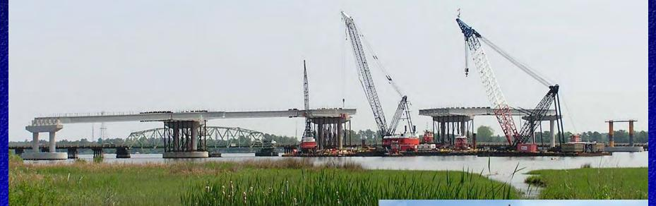
Seven segments to form the 4 spans Girders and decks are lightweight concrete
