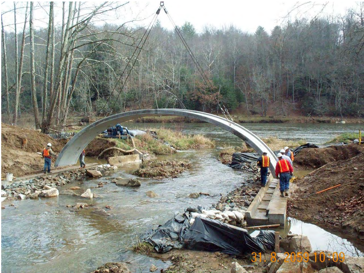
Figure 3: Installation of the first Precast arch segment
