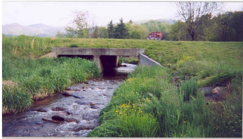
Figure 3. Culvert with Floodplain Bench
