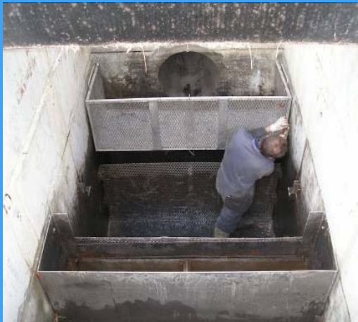
The need for confined-space entry protocols for maintenance in conjunction with inconclusive results makes evaluated proprietary BMPs unattractive.
