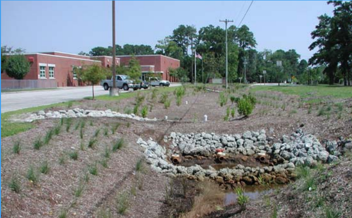
Educational rain garden installed by DOT at the Smyrna Elementary School
