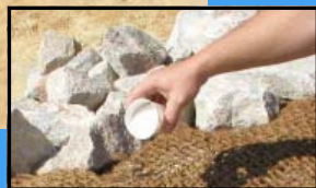
Temporary wrapped rock silt check type A dam with coir matting. Inset shows application of polyacrylamide.
