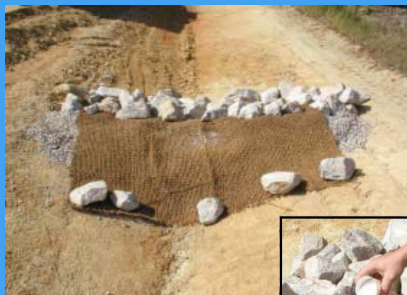
Temporary wrapped rock silt check type A dam with coir matting. Inset shows application of polyacrylamide.
