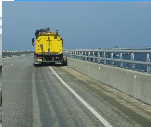
DOT implements Post-Construction BMPs for discharges to sensitive waters, including bridge stormwater collection systems (left) and sweeping (above)
