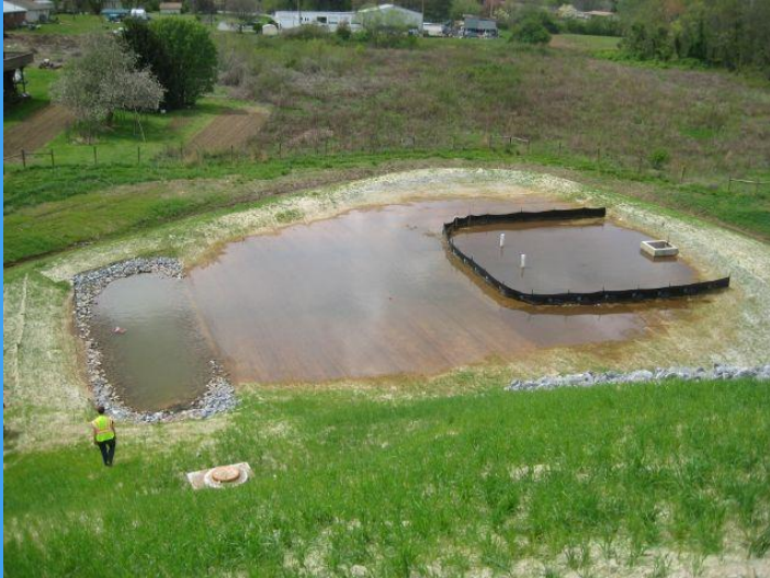
Filtration basin constructed along US 64 at the Hiwassee River
