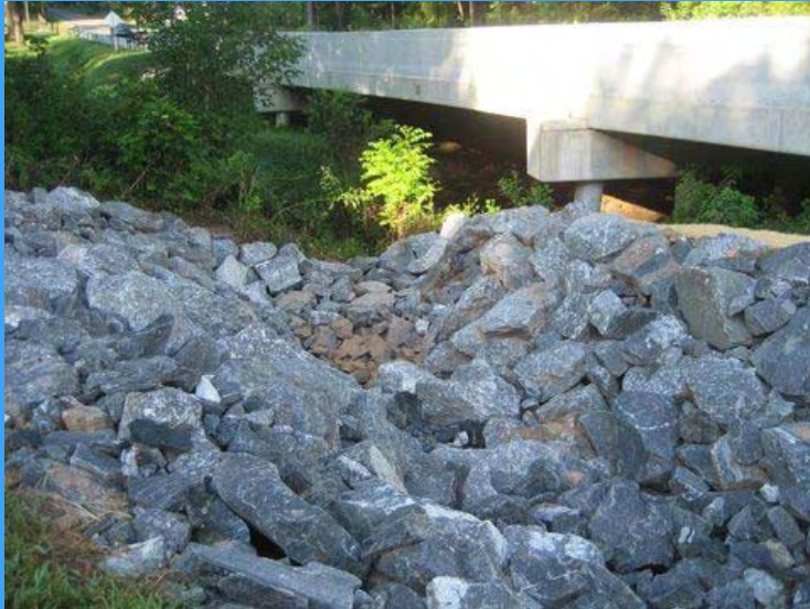
Stream Bank Drop Structure at Lee Cline Road and Cline Creek North
