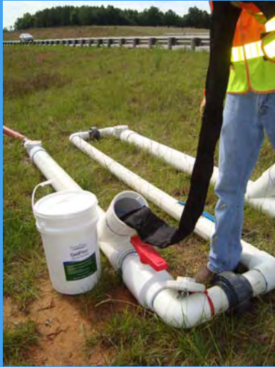
Biopolymer socks being inserted into applicator
