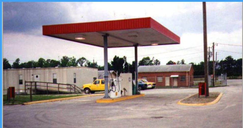
Typical DOT Fuel Station with covered canopy and fuel dispensing island. Covered canopies at DOT fuel stations provide protection of the refueling area from stormwater runoff. Fuel Station design recommendations are included in the IRMA Guidance Manual
