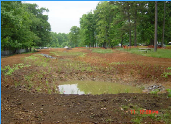
Lake Norman Rest Area Stormwater Wetland under Construction
