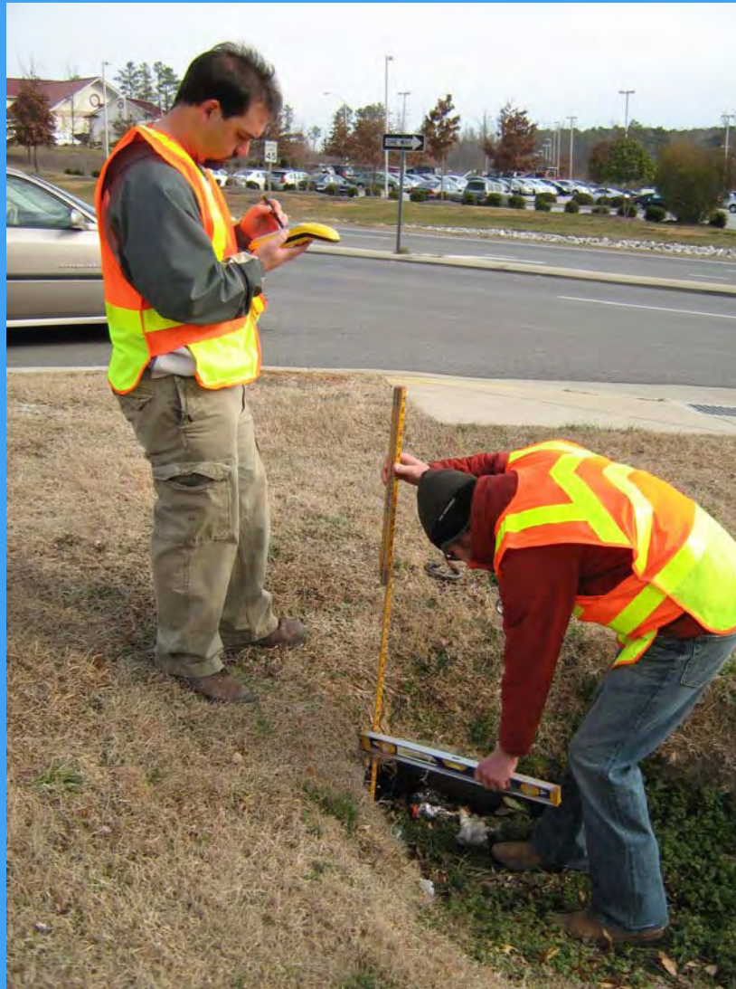
Field Staff measuring the invert of a pipe during Field Inventory Protocol testing
