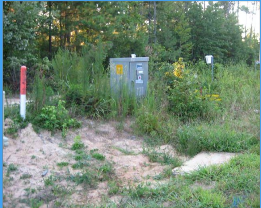
Encroachments on the ROW from the installation of third party utilities can affect NCDOT's drainage system
