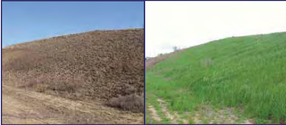
Left photo: Eroded slope before stabilization Right photo: Slope after compost seeding treatment
