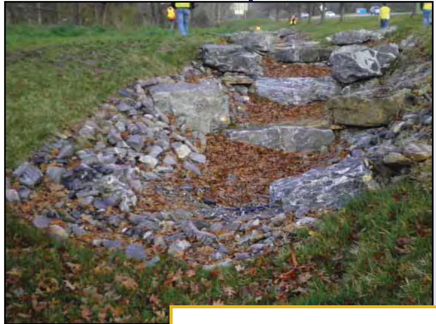
BFC system installed in an NCDOT right-of-way to treat stormwater runoff
