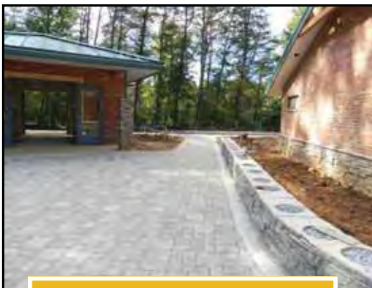
Permeable pavers installed at a rest area in McDowell County
