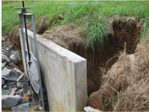
Before repairs - significant scouring around the outlet structure
