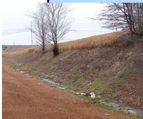
Prior to compost seeding, vegetative coverage was not well established on this slope in NCDOT's Division 2
