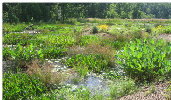
Stormwater wetlands remove a variety of pollutants by temporarily storing stormwater runoff in shallow pools
