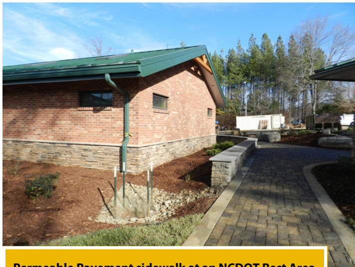
Permeable Pavement sidewalk at an NCDOT Rest Area facility in Division 13
