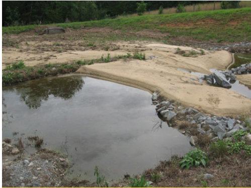
Before repairs - significant sediment build-up occurring in the HSB
