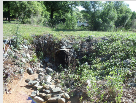
Erosion and scouring seen in the drainage system at Paw Creek prior to the BMP upgrade (left)
