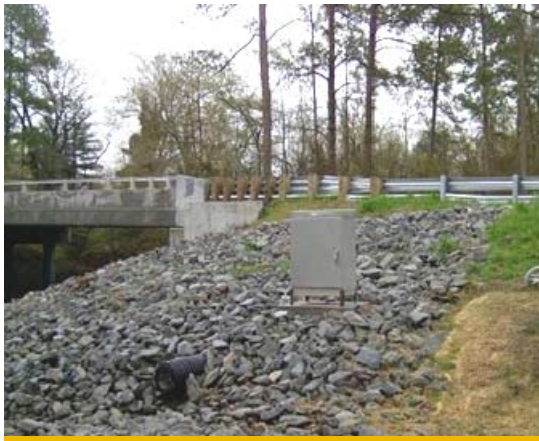
Stabilizing embankments and drainage ditches
