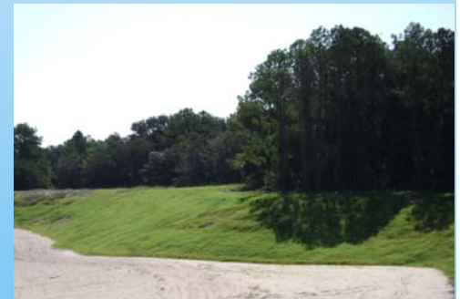
Stabilizing spoil material using compost seeding
