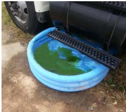
Example of a typical spill response on NCDOT right-of-way (ROW) when fuel or antifreeze leaks from a tractor trailer as a result of an accident. Spill response measures are deployed (such as this containment pool used to capture the leak); NCDOT Division personnel record the spill following IDDEP procedures and subsequently notify NCDENR
