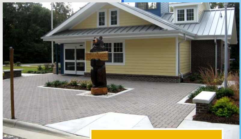
Permeable pavers installed at rest area in Washington County
