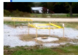
Before and after views of the new Fuel Station constructed at the new Graham (Tuluja) CMY
