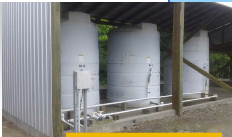
New covered containment constructed for salt brine bulk storage tanks at a NCDOT industrial facility
