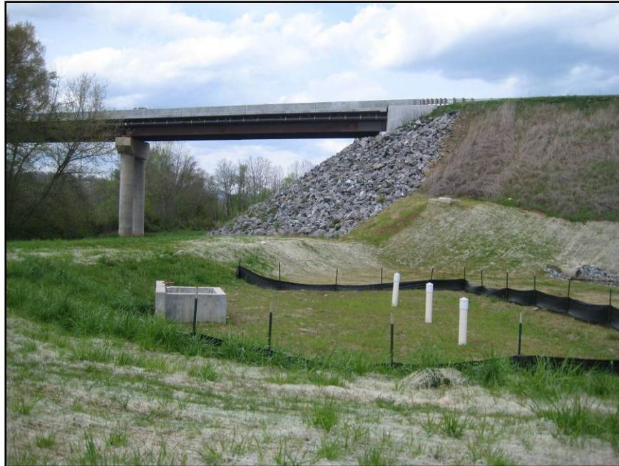
**Figure 9-2.** An example of a bridge configuration that employs common bridge BMPs: adequate ground cover and slope stabilization; as well as less frequently used BMPs: a closed deck drainage system and a downstream BMP
