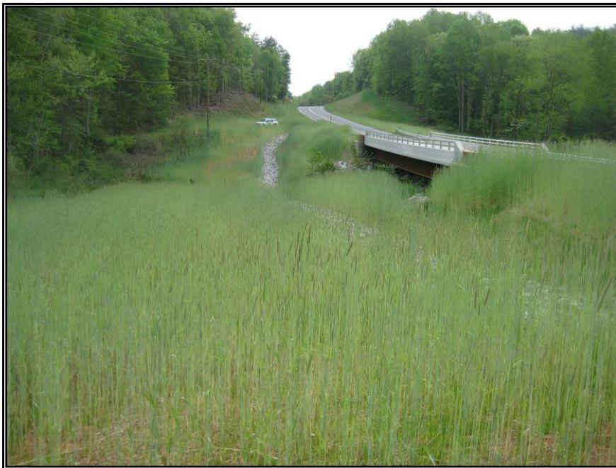
**Figure 9-1.** An example of a bridge configuration that employs some common bridge BMPs: dense ground cover, integrated road and bridge drainage conveyances
