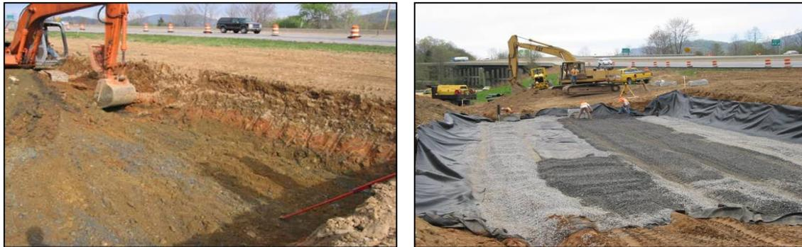
**Figure 2-6.** Bioretention basin during construction
