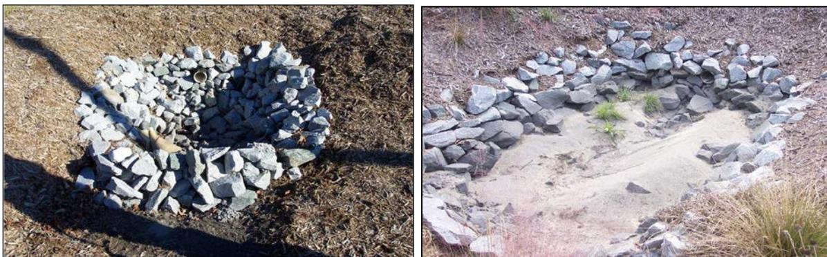
**Figure 7-5.** Maintained forebay (left) and forebay in need of sediment removal (right)
