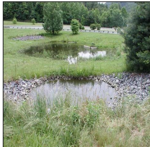
**Figure 7-1.** Riprap-lined forebay upgrade of a dry detention basin
