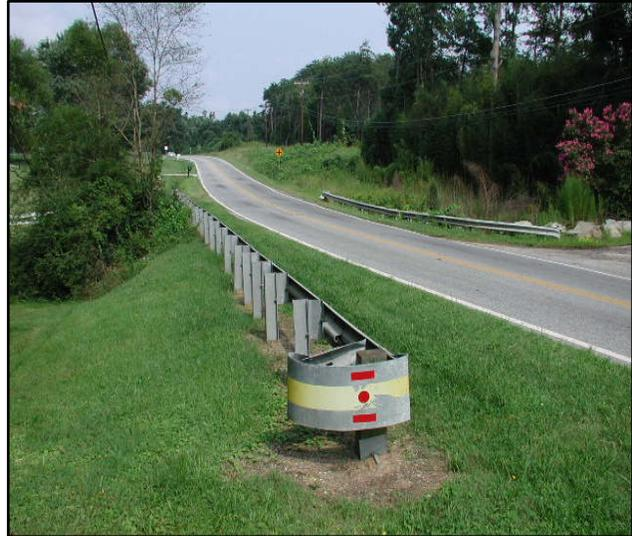
**Figure 14-1.** Typical filter strip along a roadway shoulder section
