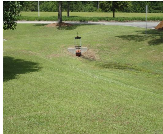
**Figure 8-1.** Typical hazardous spill basin
