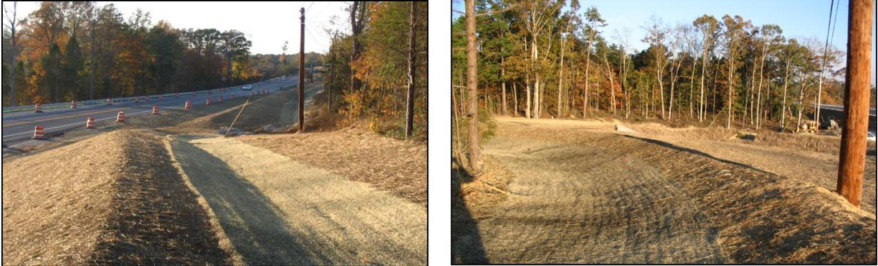
**Figure 6-6.** Swales before vegetation is established
