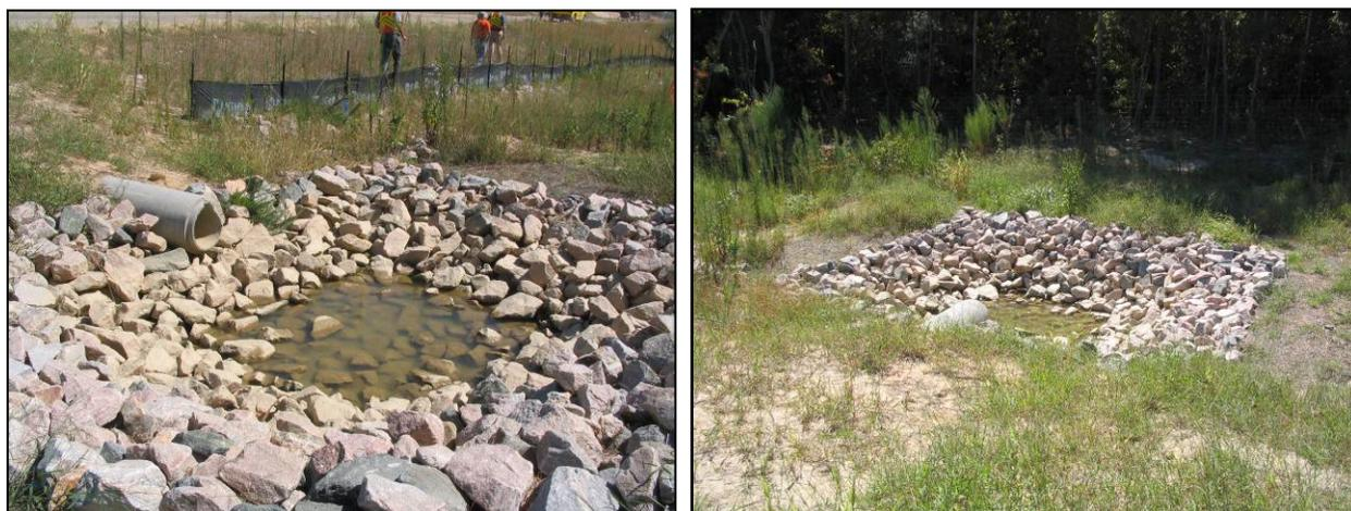
**Figure 4-1.** Preformed scour holes in a linear highway application
