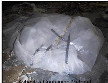
Asbestos Containing Material placed in plastic bags
