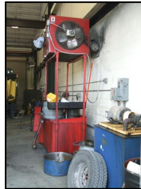
Used oil heater located in an NCDOT Equipment Shop
