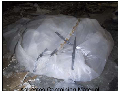
Asbestos Containing Material placed in plastic bags
