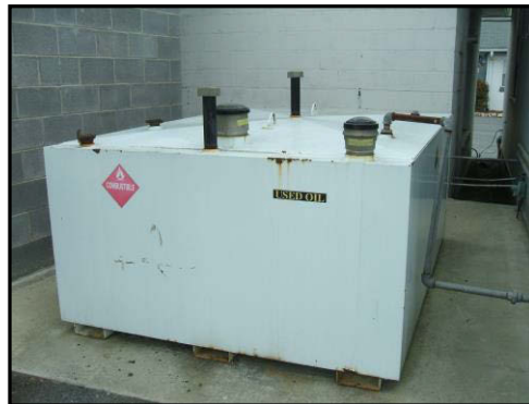
Used oil AST is double-walled
