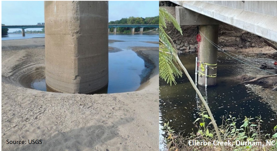
Field Monitoring Using Fiber-Optics Distributed Temperature Sensing (FO-DTS)
