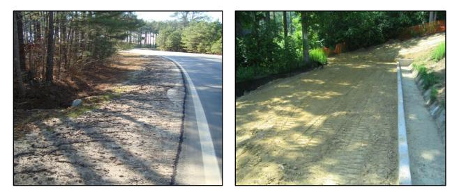
Figure 14-6. Filter strips prior to vegetation establishment
