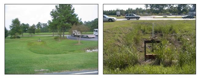
Figure 8-4. A hazardous spill basin at a rest area (left) and in a linear highway setting (right)
