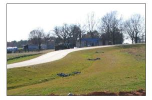
Figure 6-1. Swale with water quality rock check
