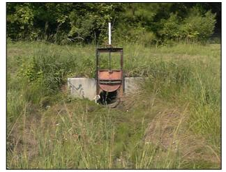
Figure 8-5. A sluice gate in a hazardous spill basin
