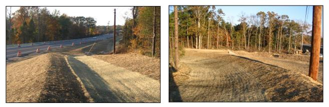
Figure 6-6. Swales before vegetation is established
