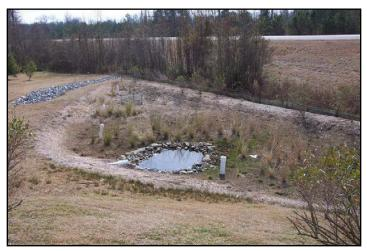
Figure 7-4. Forebay with bioretention basin
