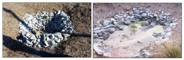
Figure 7-5. Maintained forebay (left) and forebay in need of sediment removal (right)
