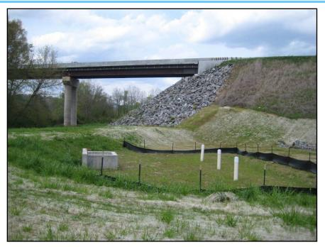
Figure 9-2. An example of a bridge configuration that employs common bridge BMPs: adequate ground cover and slope stabilization; as well as less frequently used BMPs: a closed deck drainage system and a downstream BMP
