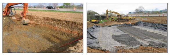
Figure 2-6. Bioretention basin during construction
