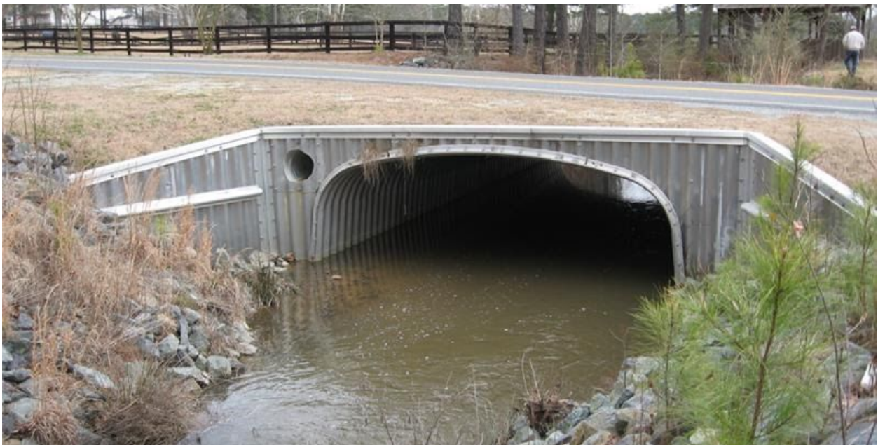
ABC w/ Corrugated Metal Headwall
