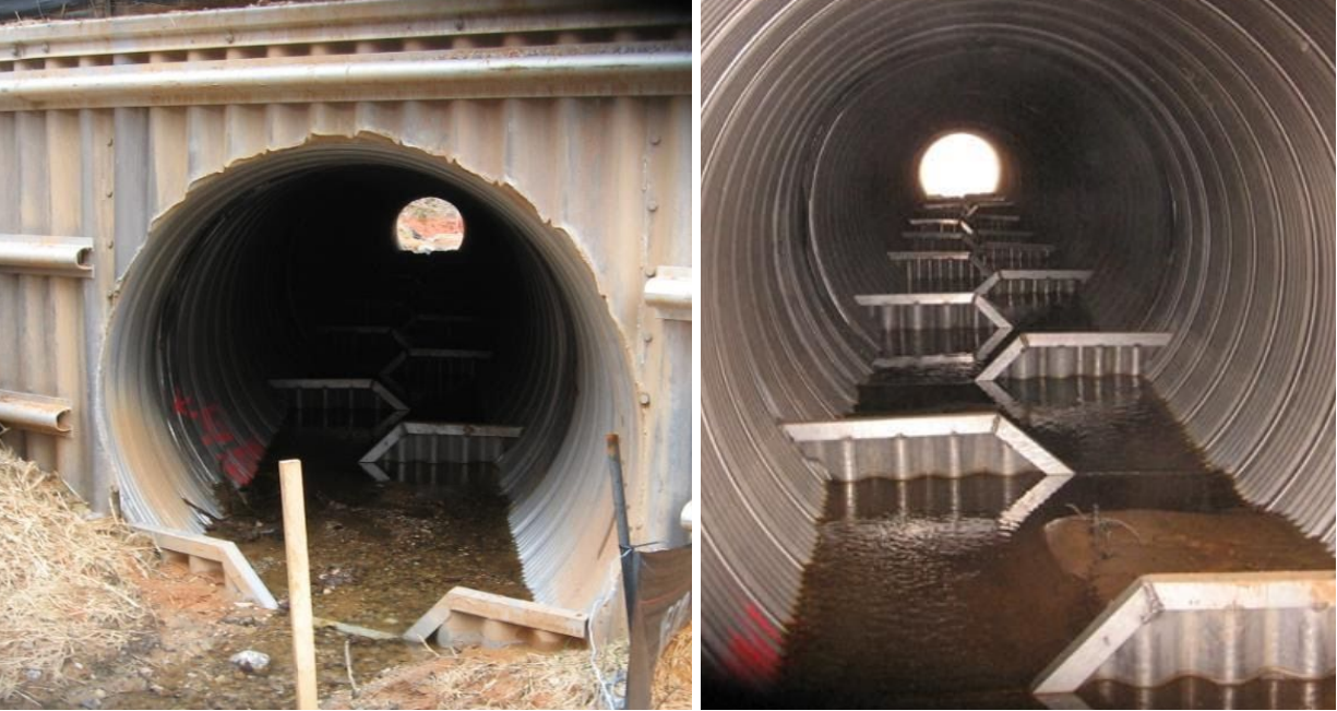
CMP with Metal Sills (at entrance) and Baffles (inside culvert)
