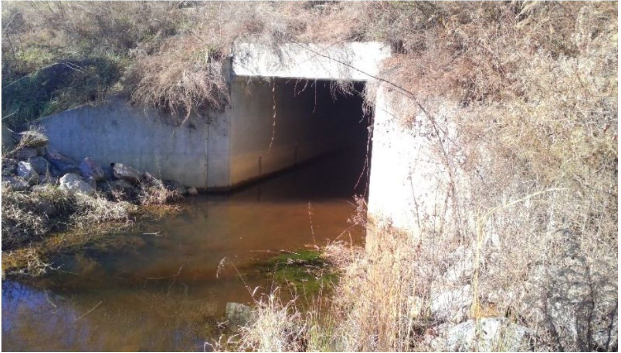
Single Barrel RCBC w/ Headwall
