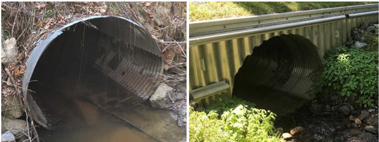
Projecting CMPA (left) and CMPA w/ Corrugated Metal Headwall (right)
