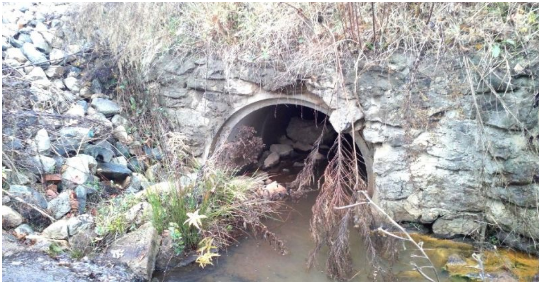
Stone Headwall for RCP
