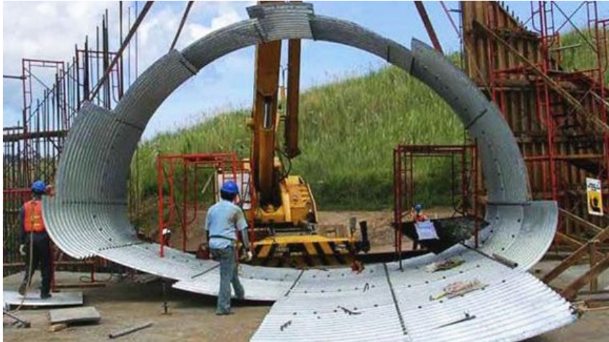
Structural Plate Arch being constructed in the field
