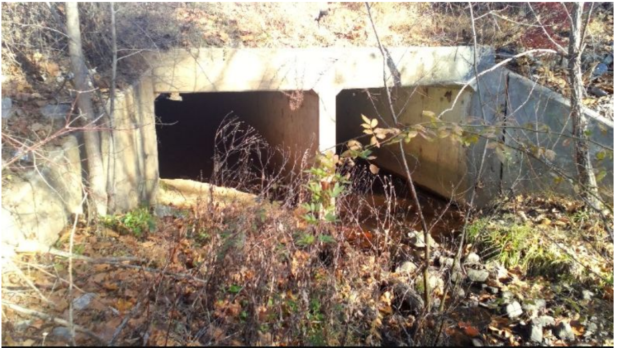
Dual Barrel RCBC with Headwall
