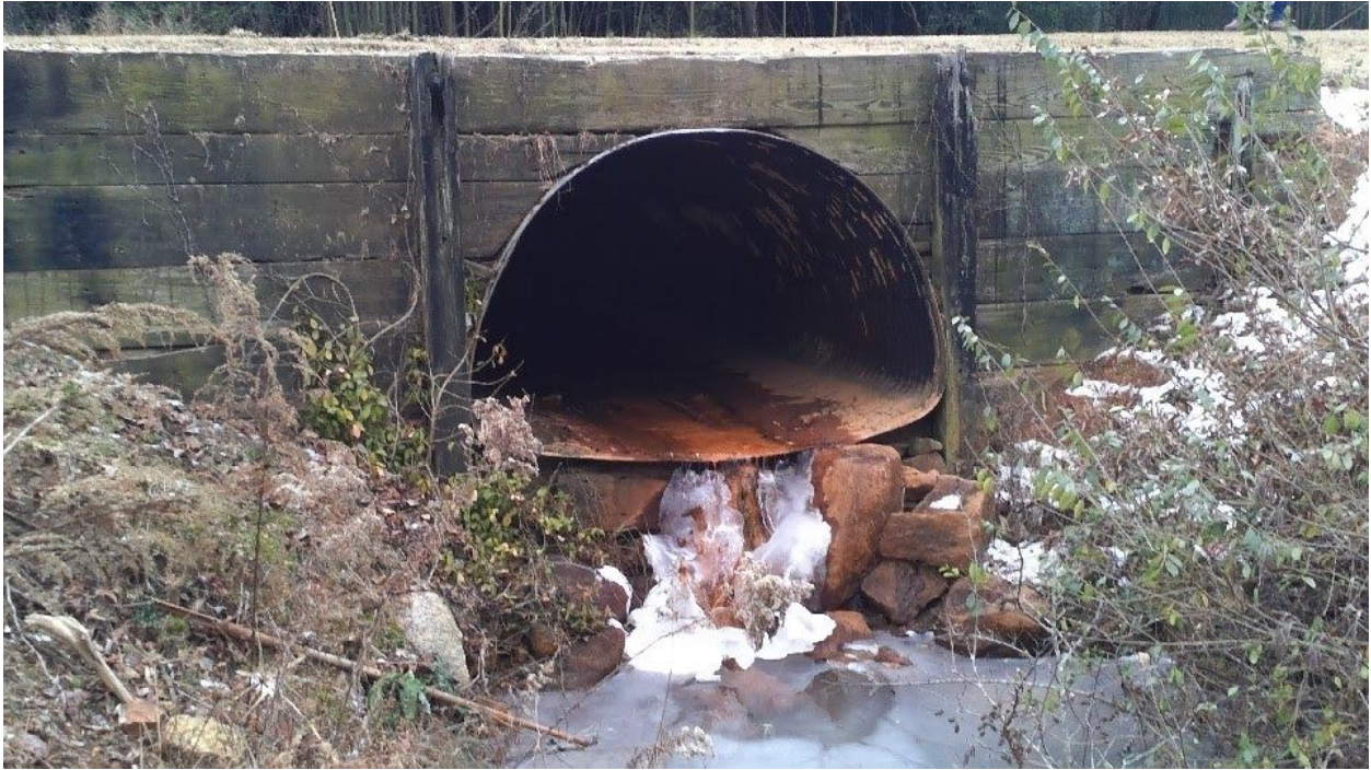
Timber Endwall for CMPA (outlet)
