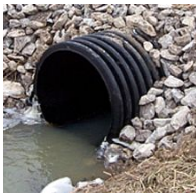
Projecting HDPE culvert
