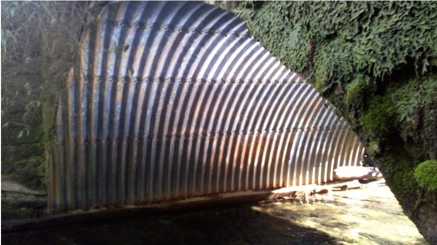
Bottomless Structural Plate Arch Inlet (note bolted plates)
