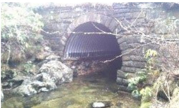
Bottomless CMPA Culverts with Stone Headwall (left) and Concrete Headwall (right)
