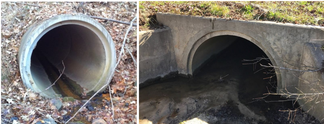
Projecting RCP (left) and RCP w/ Concrete Headwall (right)
