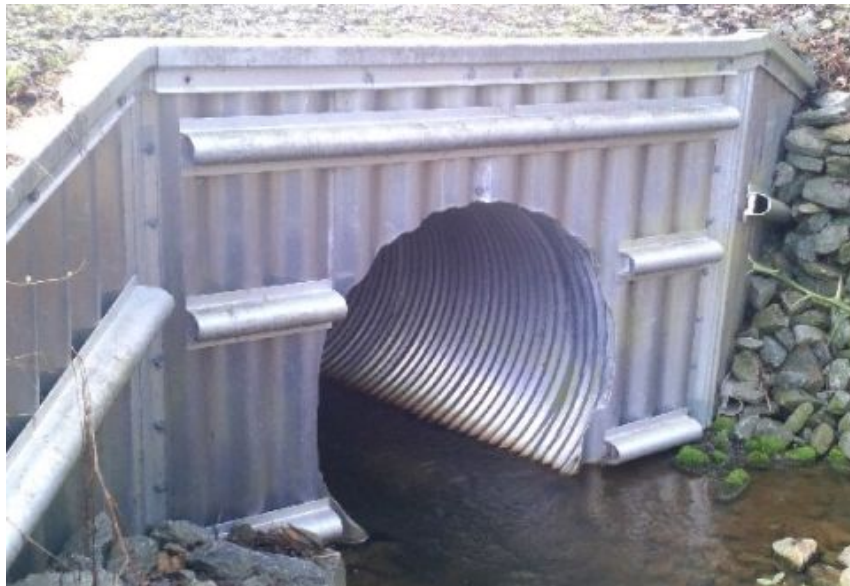
CMP w/ Corrugated Metal Headwall
