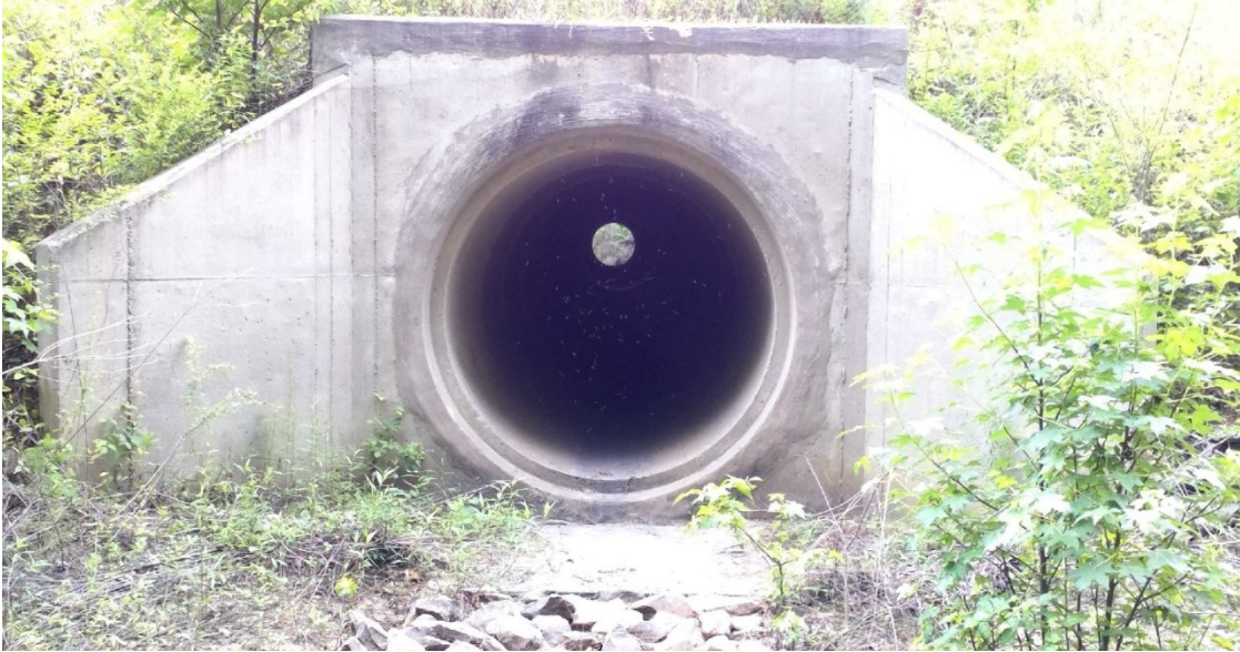
Concrete Headwall with wing walls for RCP
