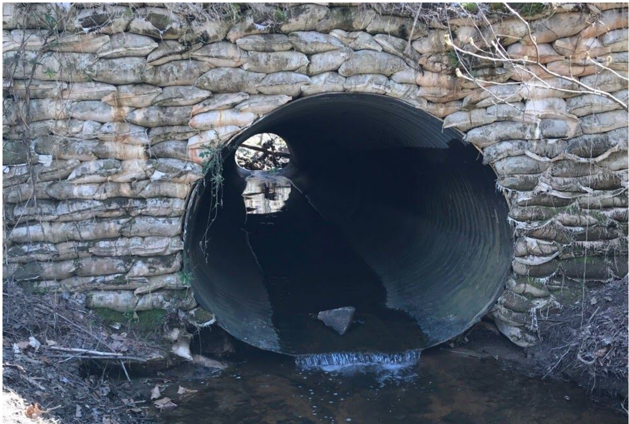
Sandbag Endwall for CMPA (outlet)
