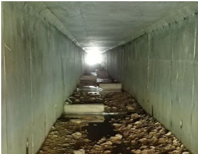
Concrete Baffles in RCBC
