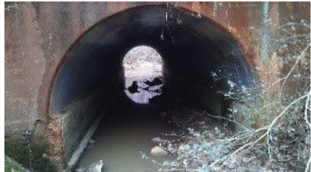
Bottomless CMPA Culverts with Stone Headwall (left) and Concrete Headwall (right)
