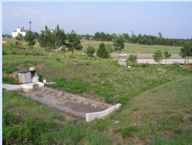
Figure 2.2-9: A filter strip that receives overpass runoff at Hwy 42 and I-40 in Johnston County, North Carolina (Wu and Allan, 2006).
