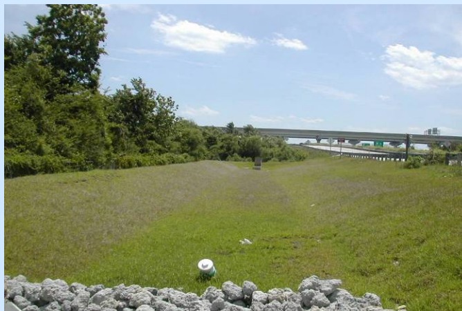
Figure 2.2-10: A filtration basin treating runoff from a concrete bridge over the Trent River in New Bern, North Carolina (Line, 2006).
