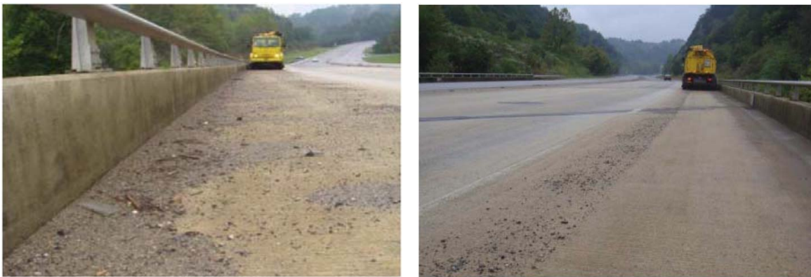
Figure 3.3-5: Bridge deck before sweeping (left) and after sweeping (right).
