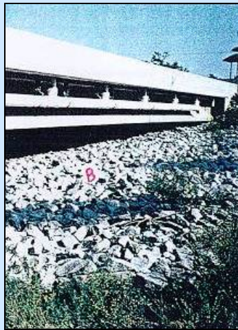
Figure 2.2-8: Stormwater spoil area near the Isle of Palms Connector in South Carolina (Ross and Leitman, 1994).
