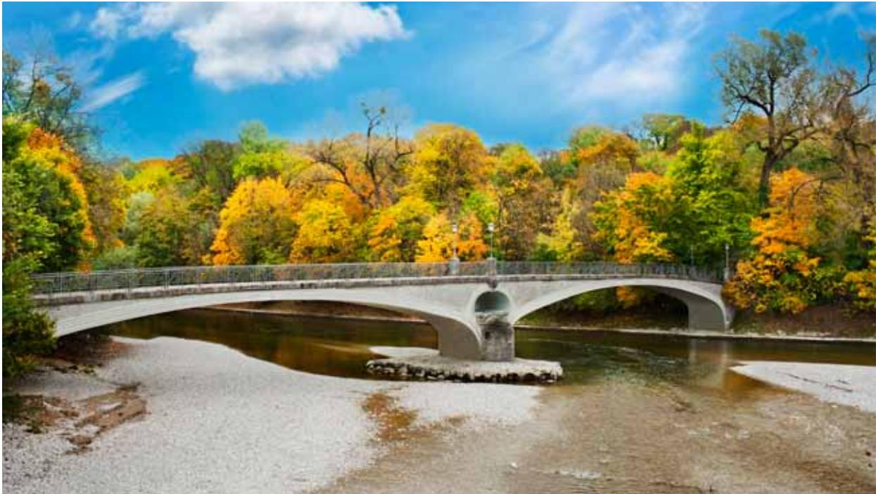
*This bridge in Munich, Germany has two long, flat arches that are supported by a central column. The stone pattern on the bridge walls, the smooth lines of the arches, and the open rail all combine to define the visual character of the bridge. Image courtesy DepositPhotos.com.*
