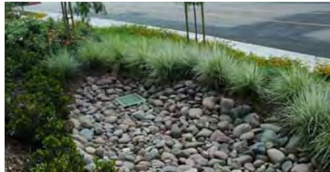
Gravel is used to slow down stormwater runoff in this bioswale, and the plants filter sediment and pollution runoff. Image courtesy EDAA.
