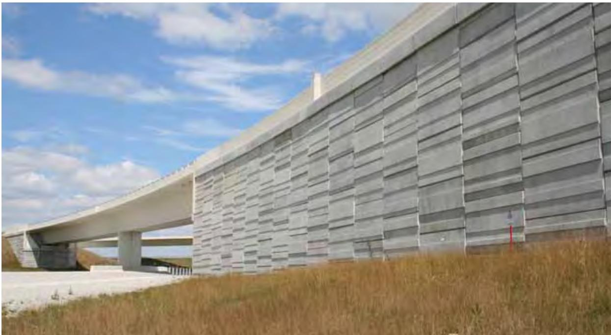
*The retaining walls that make up the abutments for this bridge along I-70 near the Indianapolis Airport are constructed of reinforced earth MSE precast retaining wall. The smooth texture and white color of the bridge and railings visually fit with the light to medium gray panels that look a bit like slate. Image courtesy INDOT.*
