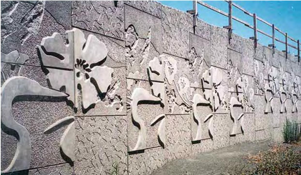
*This concrete retaining wall by Braaksma Design Inc uses custom images created from off-the-shelf textures.*
