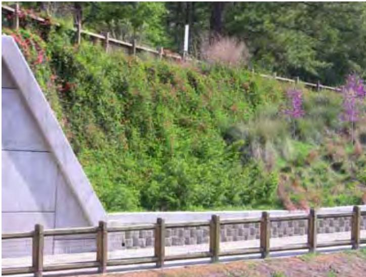
*This is another example of using native materials to create a green wall along the grade separation of the roadway and a multipurpose trail. Image courtesy EDAW.*
