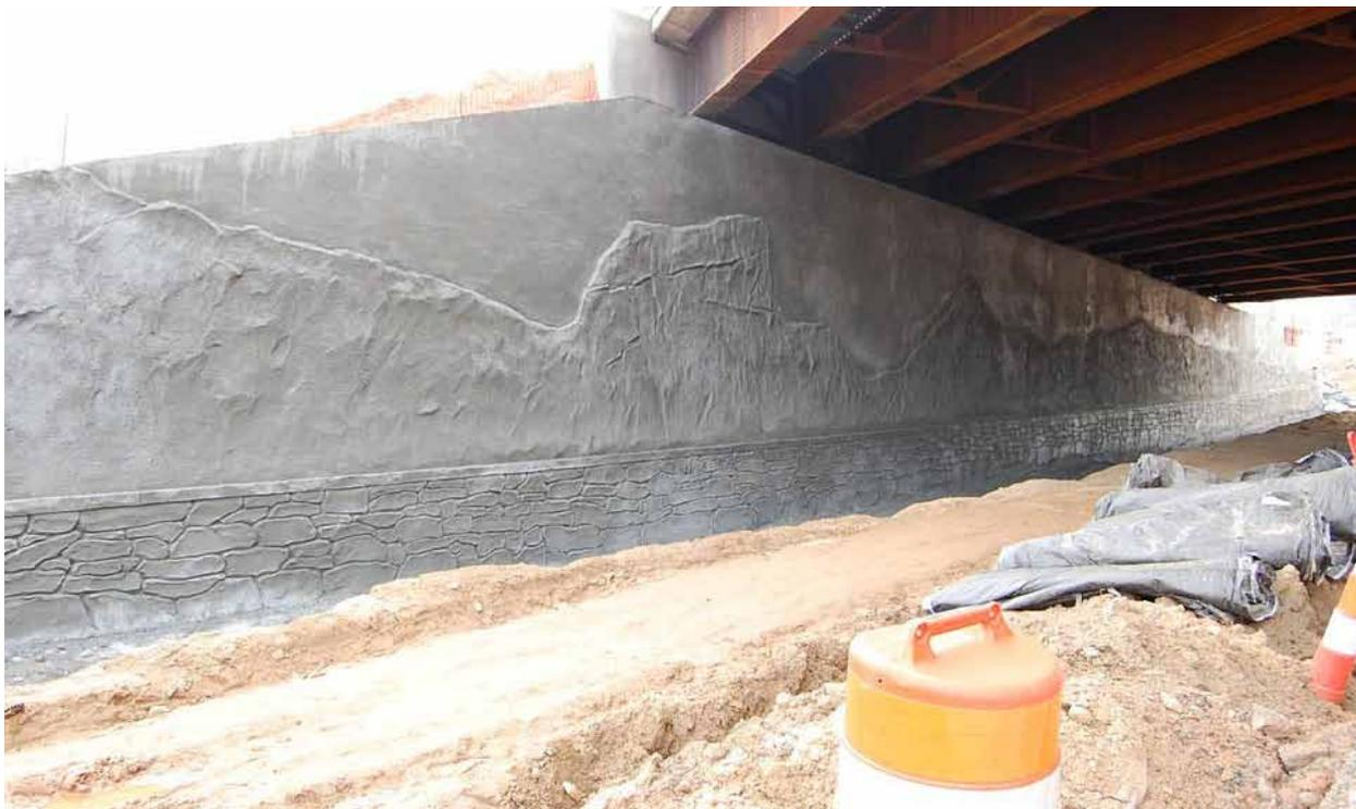
*NCDOT is replacing both bridges at Interstate 40 Exits 105 on Sterling Street and Exit 104 on Enola Road. This provided an opportunity to improve visual character of the bridges. Enhancements at Exit 105 include two murals on the underpass walls, stone treatments to the bridge rails, and stone treatment of a retaining wall on the westbound off ramp. Images courtesy NCDOT.*
