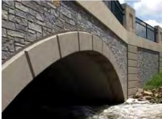
*This wall uses a minnehaha blend form liner to create the appearance of stone. Image courtesy Customrock.*
