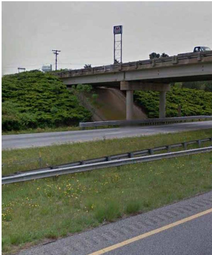
*These images show Standard bridge abutments (very top & right) that are poured-in-place concrete that stabilizes the slopes, with plantings along the sides, The image above shows a Standard concrete retaining wall along a roadway. Image courtesy James Sipes.*
