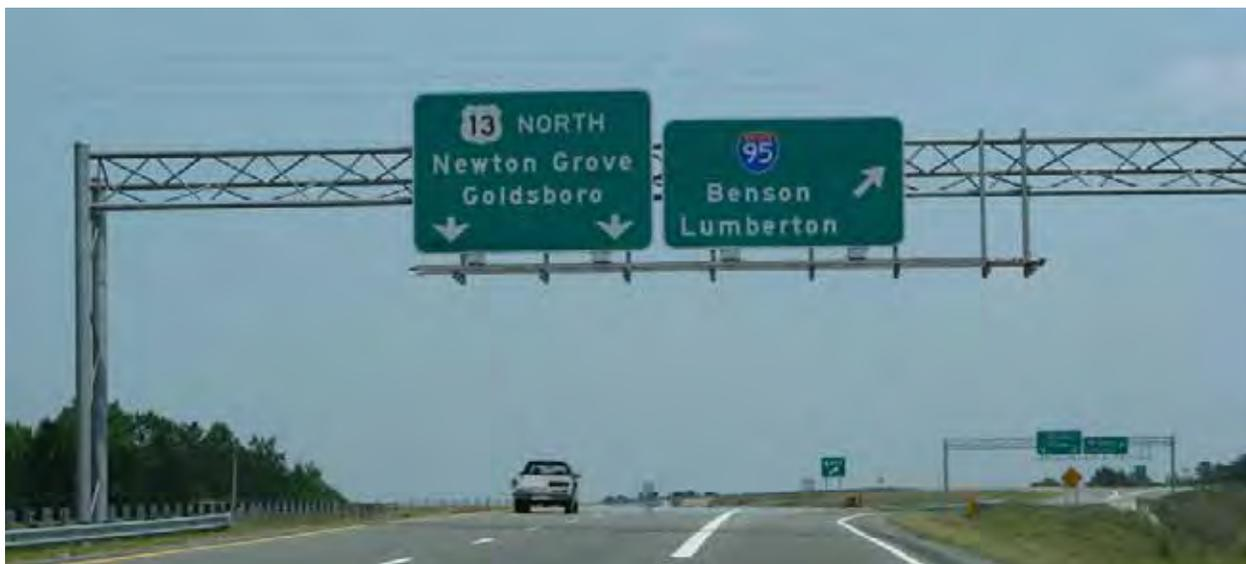
*A standard sign gantry on I-295 is used to support directional signage for 13 North and I-95. The small size of the metal components, openness of the horizontal elements, and light gray color of the structure helps reduce the visual impact of the gantry. Image courtesy NCDOT.*
