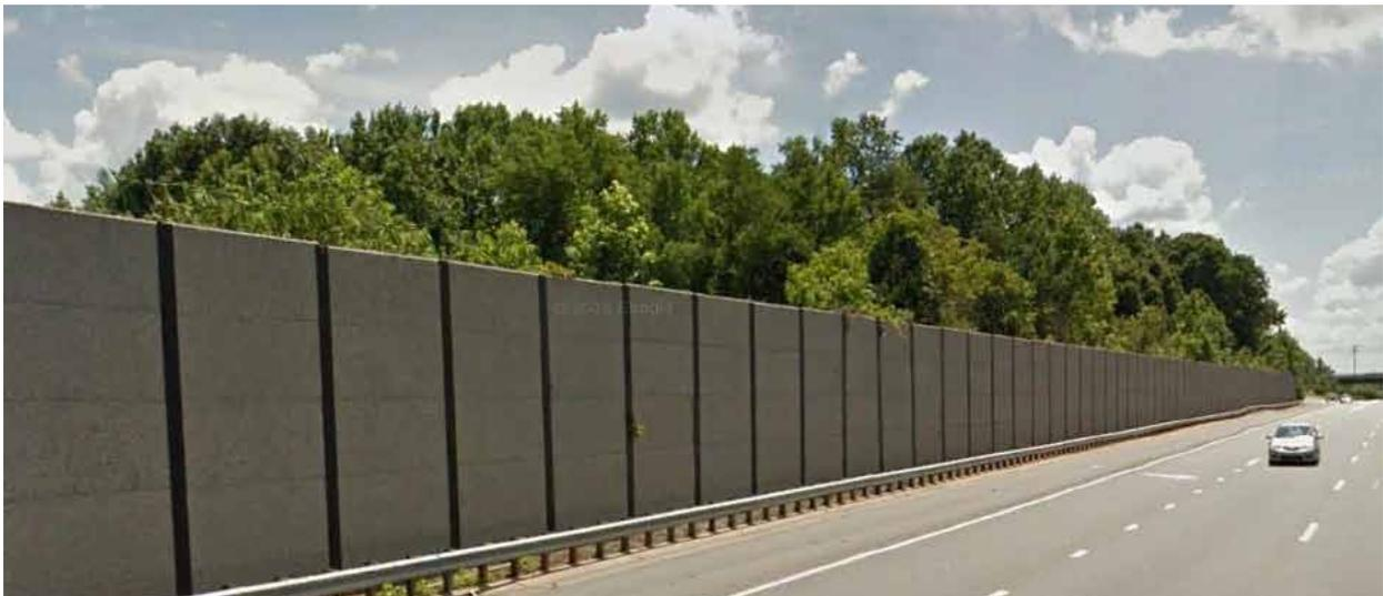
*These are examples of Standard Noise Walls used along North Carolina roadways. Both use a pier and panel approach for wall construction. Images courtesy NCDOT.*
