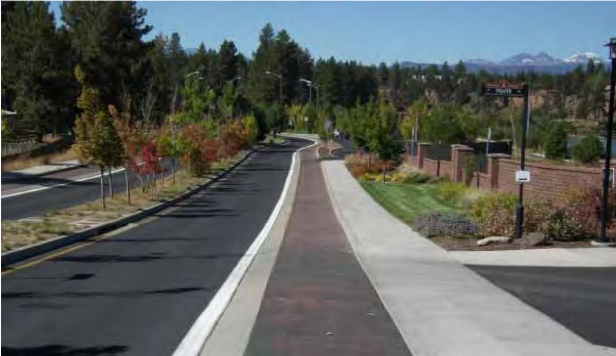
*Along US Highway 97 in Bend, Oregon, are stained walk/bike trails, raised medians with native plant materials, a meandering road geometry to maintain a pedestrian scale, and lighting for security and safety. Image courtesy Oregon DOT.*
