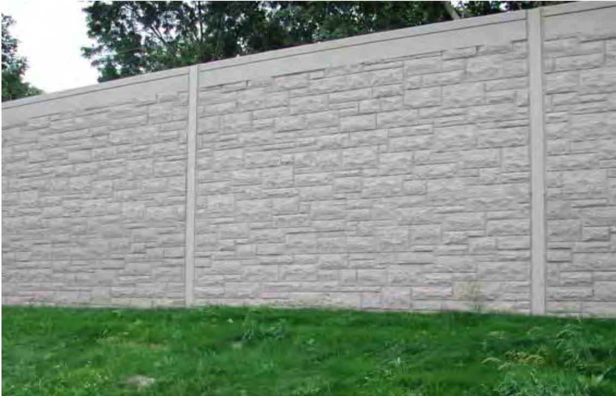
*This standard NCDOT wall includes steel pilings, an ashlar stone pattern created with form liners, and a faux top created by a smooth surface along the top of the wall. Image courtesy James Sipes.*
