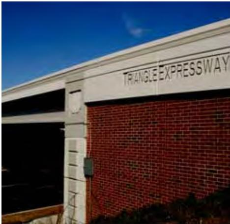
*View of a bridge abutment that is part of the Triangle Expressway Toll Road. The brick and light colored concrete defines the visual character of elements that are part of the expressway. Image courtesy NCDOT.*
