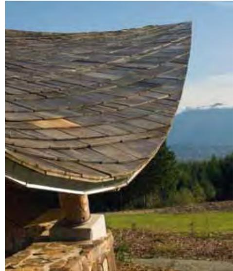
*The shelter at Snoqualmie Point has a free-flowing curved roof that is a visually dominant element. Mt. Si, Washington, is in the background. Image courtesy Jones + Jones.*
