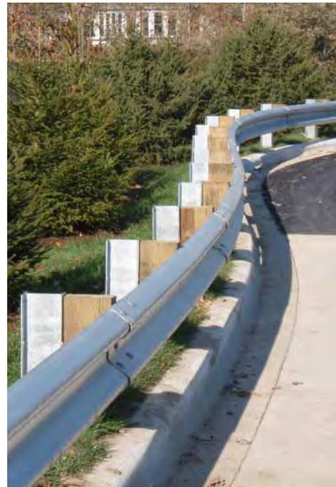
This image shows a typical steel guardrail. Image courtesy FHWA.
