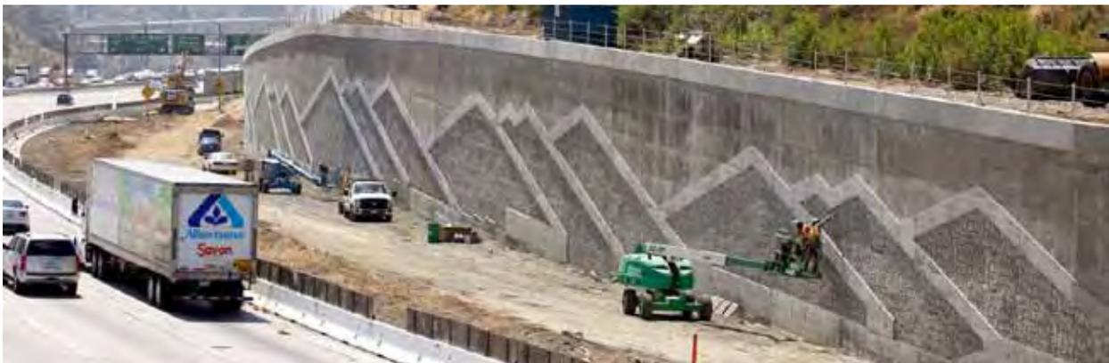
*This large retaining wall uses a mosaic of mountain peaks created with form lined concrete to add visual interest and break up the perceived scale of the wall. Image courtesy FHWA.*
