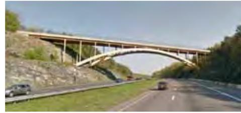
*The Ridge Road Bridge over I-70 in Frederick County, Maryland, serves as a visual landmark because of the strong, simple lines of the top deck and support columns, and the curved arch of the bottom support. The bridge crosses I-70 at an angle, so the bridge is shown with foreshortening. Image courtesy FHWA.*
