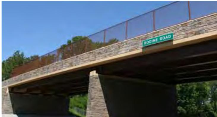
*Fieldstone patterns are used for piers, rails, and abutments of the Bodine Road, which crosses the Pennsylvania Turnpike. Image courtesy James Sipes.*
