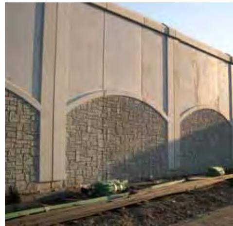
*Construction for this concrete retaining wall is nearing completion. Form liners were used to create the patterns. Image courtesy FHWA.*
