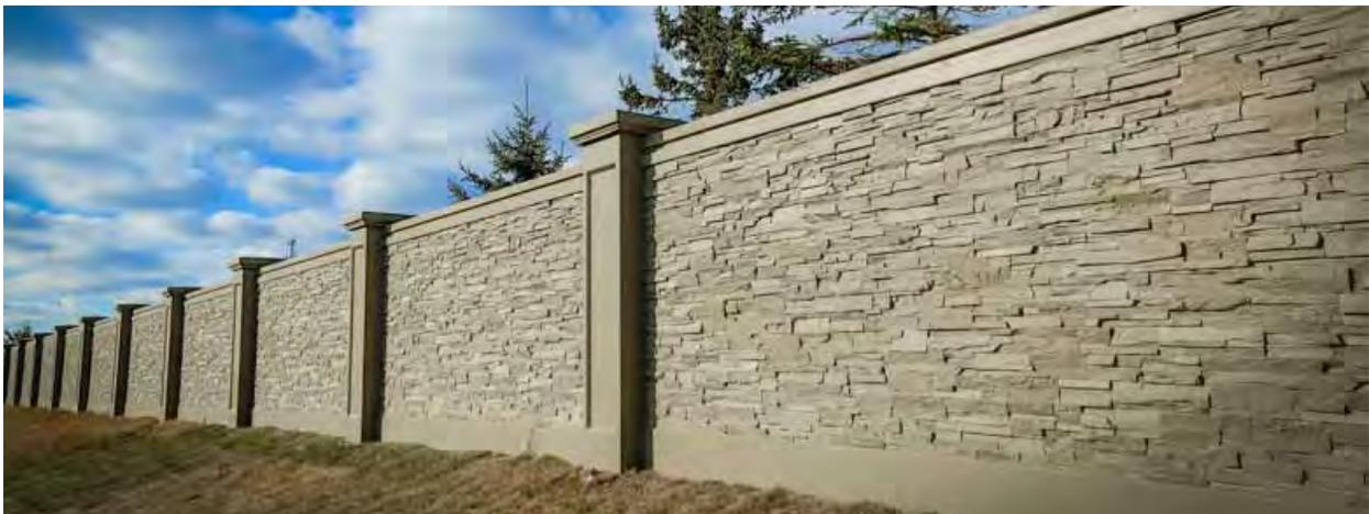
*This precast concrete noise wall uses a fieldstone pattern on the panels, a shadow box and cap on columns, and a smooth pattern for the base and cap of the panels to add visual consistency and continuity. All of the components are a light grey, which helps reduce the visual dominance of the wall. Image courtesy James Sipes.*
