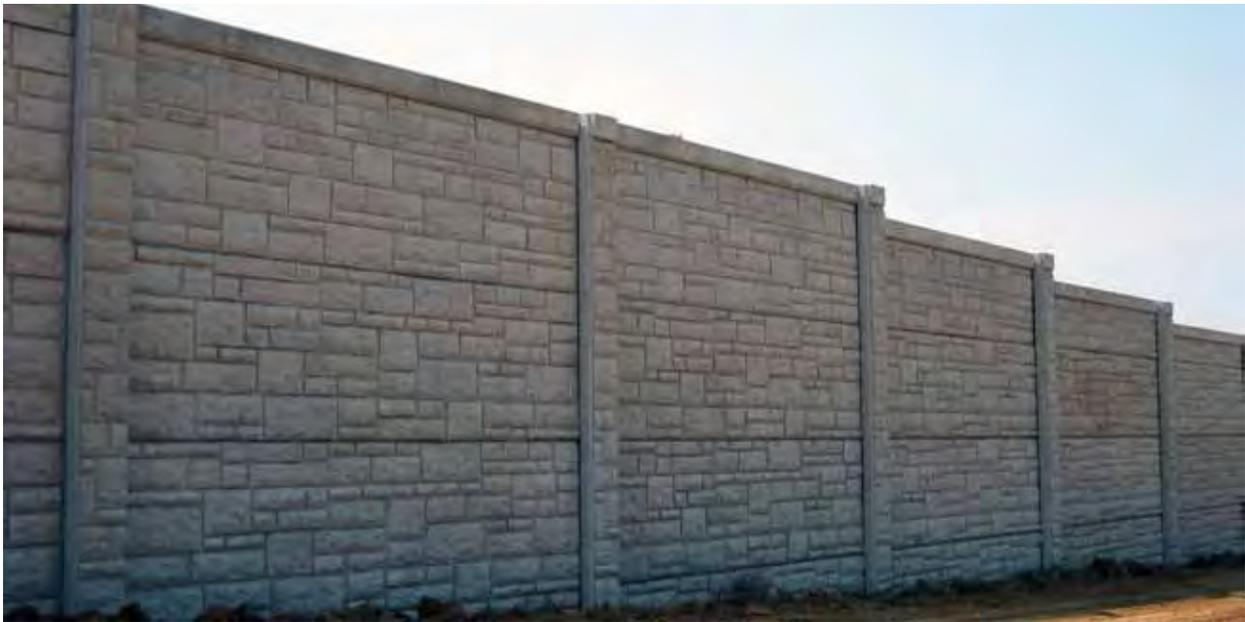
*This ashlar stone finish noise wall includes a reflective facing. This side of the wall is on the residential side of the development. Image courtesy NCDOT.*
