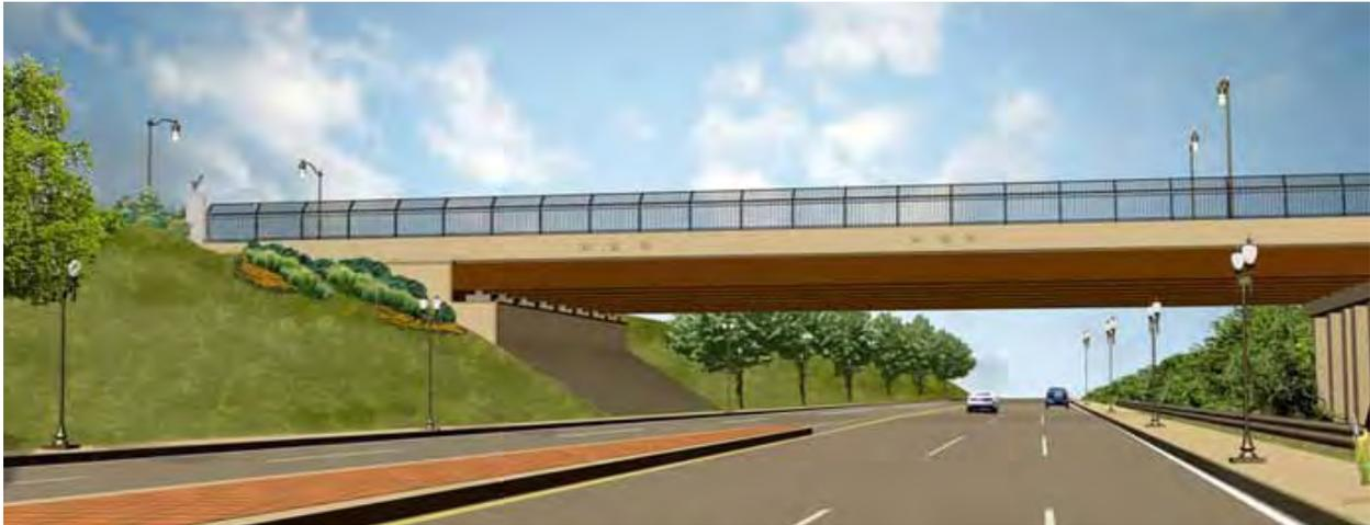
*This simulation of the 9th Street Bridge in Washington, DC, uses darker colors for the girders that extend across the roadway as well as pigmented or painted concrete elements. Image courtesy Creative Design Resolutions.*
