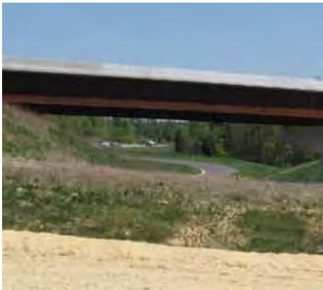
*The flyover ramp from I-74 East to I-85 North uses a simple steel plate girder design with concrete for support. Image courtesy NCDOT.*
