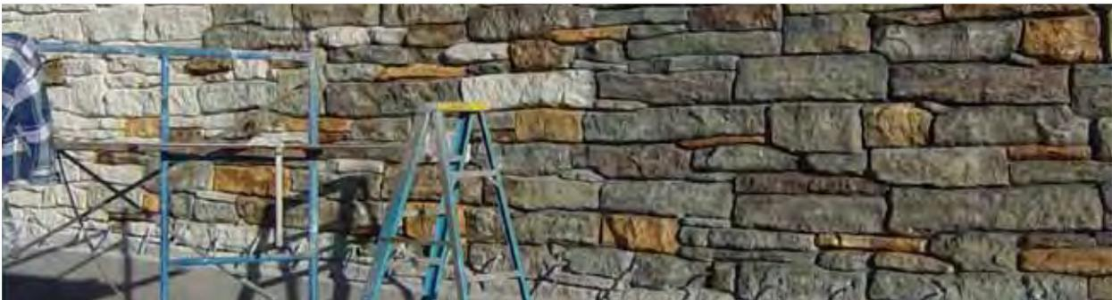
*This image shows how a wall created with a form liner is being stained by hand to create a more realistic appearance of the stone. Image courtesy NCDOT.*
