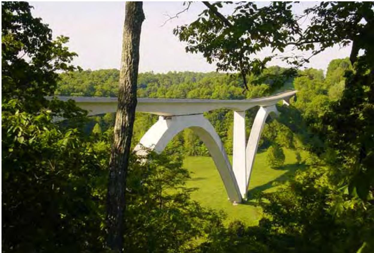
*The Natchez Trace Parkway Bridges is a double-arch bridge that spans across Highway 96 near Nashville, Tennessee. It's located at mile marker 438 on the Natchez Trace Parkway. The bridge was completed in 1994, and is the first segmentally constructed concrete arch bridge in the United States. Image courtesy FHWA.*
