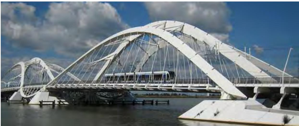
*The segmented appearance of the Enneus Heerma Bridge is based on the skeleton of a crab. The wavy pattern of the bridge represents water. The arches were pre-assembled arches and floated in on pontoons, and then lifted by cranes. Image courtesy Wikipedia Commons.*
