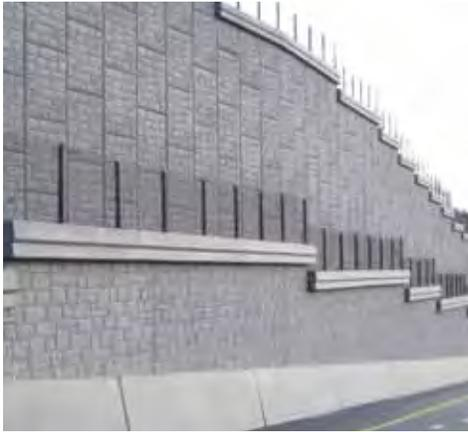
*Retaining walls along I-405 through Renton, Washington, are constructed of precast Mechanically Stabilized Earth (MSE) wall panels. The smooth texture of the horizontal caps and base provide a level of contrast from the stone panel texture. Image courtesy WSDOT.*
