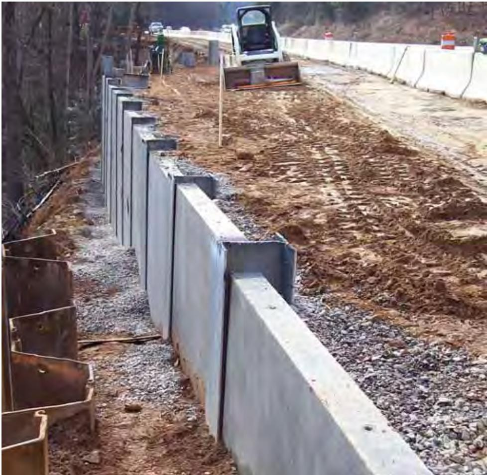
*These retaining walls constructed of steel piers and precast concrete panels are used to stabilize slopes along North Carolina roadways. Emphasis is more on functionality than aesthetic appeal. Image courtesy NCDOT.*
