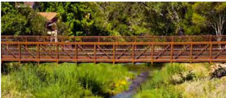
*This corten steel bridge provides pedestrian access from one side of the creek to the other. The dark color of the steel bridge helps in visually blend with surrounding landscapes. Image courtesy DepositPhotos.com.*
