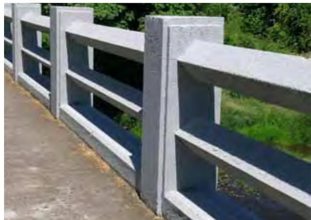
*Massive geometric concrete rails are used on the Brownsville Bridge, Texas. Image courtesy FHWA.*
