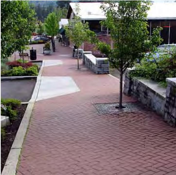
*This pedestrian walkway in Lake Oswego, Oregon, is a good example of an enhanced walk. The use of brick pavers, concrete curbs and accessibility ramps, tree grates, retaining walls, and variety of landscaping all help create a comfortable, inviting pedestrian space. Image courtesy PBIC Image Library and Dan Burden.*
