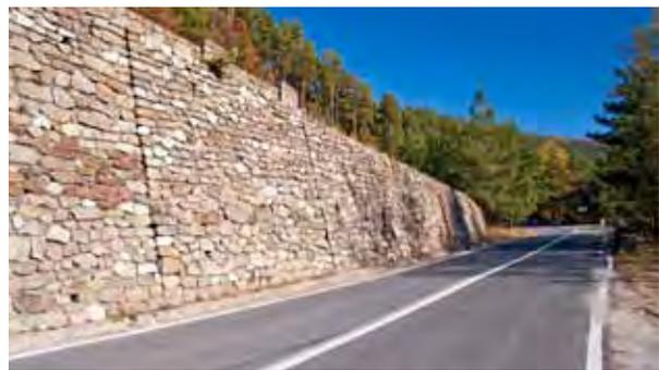
*Despite its height, this retaining wall is not visually objectionable because the stone veneer reduces the perceived scale of the wall. Image courtesy DepositPhotos.com.*
