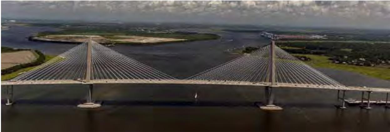
*The Arthur Ravenel Jr. Bridge, near Charleston, South Carolina, uses a cable-stayed suspension design with two diamond-shaped towers. Each tower is 575 feet tall, and the combination of towers and cables help make this a landmark bridge. Image courtesy David Oppenheimer.*
