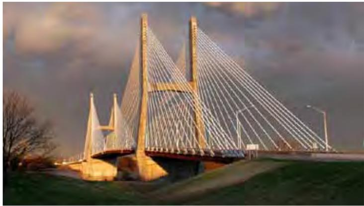
*The Bill Emerson Memorial Bridge extends over the Mississippi River at Cape Girardeau, Missouri. It is a cable-stayed bridge, and the combination of cables and the towers (or pylons) used to allow the cables to support the bridge deck create a dynamic visual image. Image courtesy Wikipedia Commons.*
