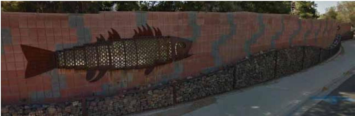
*This sound wall in Scottsdale, Arizona, is designed to be a positive visual element within the community. The wall has a curved shape that is augmented by the meandering patterns of stone encased in a metal mesh, and the diagonal pattern of the bricks in the wall help suggest the fish is moving forward. The same wall pattern is used along the length of the street. Image courtesy James Sipes.*
