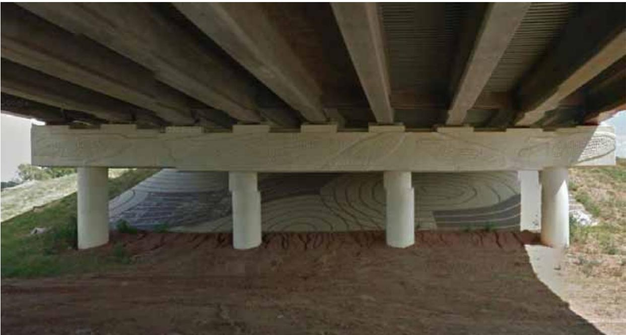
*The abutments and beam under a bridge for SR 9 over I-35 in Norman, Oklahoma, include decorative patterns. Image courtesy James Sipes.*
