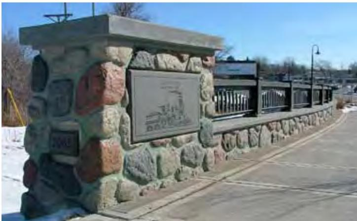
*This wall with the railroad sign includes a Minnesota fieldstone form liner pattern and metal rails. Image courtesy Customrock.*
