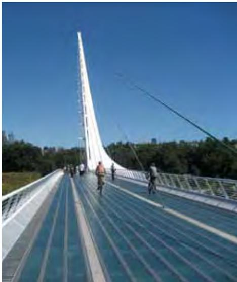
Santiago Calatrava’s Sundial Bridge is a cantilever spar cable-stayed bridge for bicycles and pedestrians that spans the Sacramento River in Redding, California. The bridge has become iconic for Redding. The tall vertical element serves as a visual focal point. Image courtesy Wikipedia Commons.
