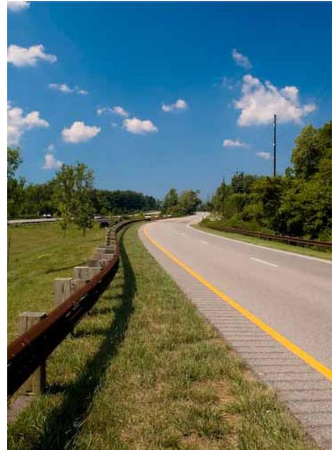
*Reinforced grass shoulders are used to reduce the visual scale of Paris Pike in Lexington, Kentucky. The shoulders can be used for emergency stops because geotechnical cell grids provide reinforcement for the soil. Image courtesy James Sipes.*
