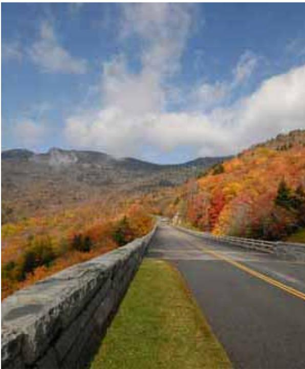
*This view of Blue Ridge Parkway shows the use of stone retaining walls, narrow shoulders, and a limited right of way to minimize impacts on the surrounding landscape. Image courtesy FHWA.*
