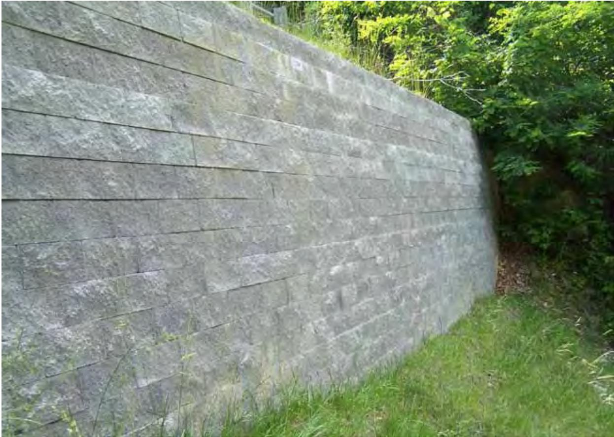
*This standard retaining wall is constructed of modular concrete blocks. Image courtesy NCDOT.*
