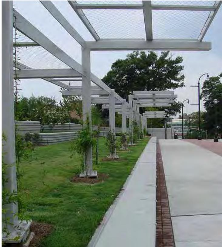
*This overhead structure provides visual interest for this overpass. The overhead trellis will eventually be covered by the vines planted at the base of each post. This will soften the impact of the structure and create a more inviting pedestrian walk. Image courtesy EDAAW.*
