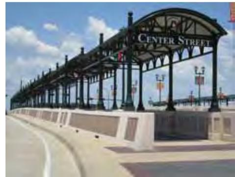
*The dark green, metal structure that extends over Center Street in Arlington provides shade for pedestrians and also provides an extra level of visual interest. Sign posts and light fixtures use a similar style. Barriers along the road are enhanced by using dark tan panels surrounded by a light gray, smooth concrete. Image courtesy James Sipes.*
