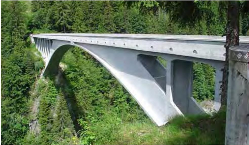
*Salginatobel Bridge is a reinforced concrete arch bridge designed by Swiss civil engineer Robert Maillart. It was constructed across an alpine valley in Schiers, Switzerland between 1929 and 1930. Image courtesy Wikipedia Commons.*
