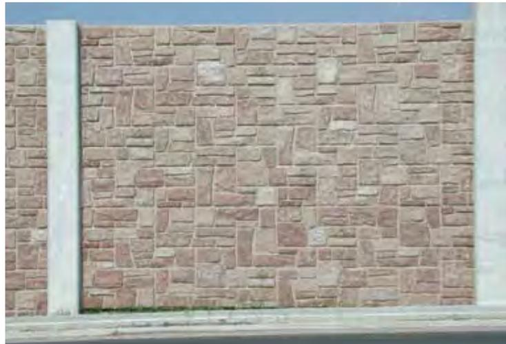
*A rustic ashlar stone pattern stained to create a darker surface is outlined by smooth concrete piers. There is no cap along the top of the wall. Image courtesy Customrock.*
