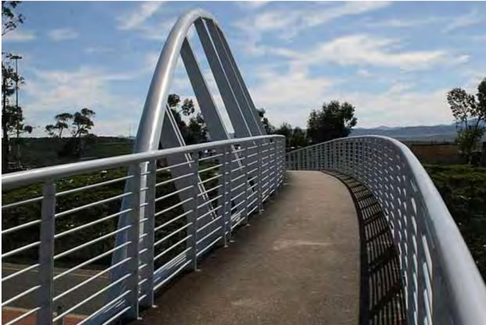
*SMEC South Africa developed a design for the Plettenberg Bay Pedestrian Bridge in South Africa that incorporated an inclined arch with a slender steel torsion box deck. The central span of 92 feet is supported by the inclined arch with the continuous back spans almost 30 feet. Image courtesy SMEC South Africa.*
