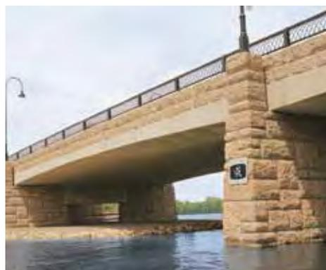
A sandstone ashlar pattern was created for this bridge using form liners. The beige color of the stone pattern contrasts with the lighter color of the bottom of the arches. Image courtesy Customrock.
