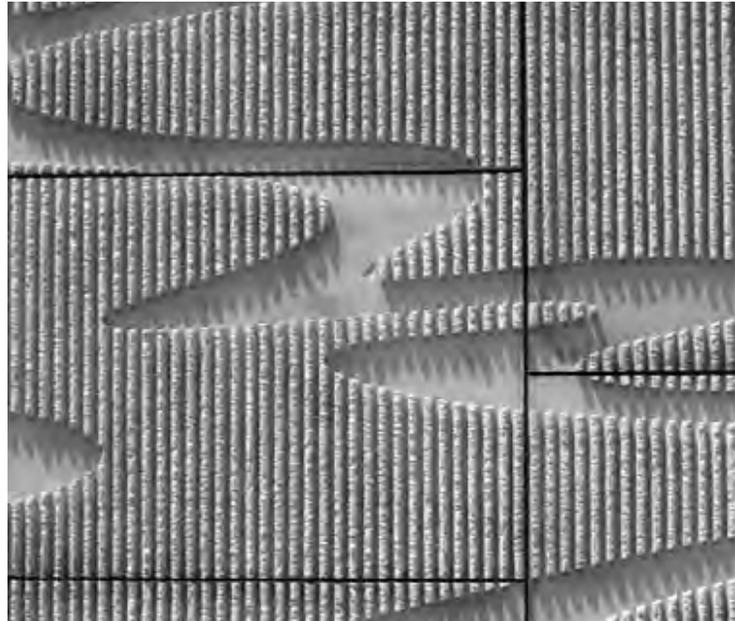
This is an example of precast concrete panels that fit together to create a wave pattern. The combination of the wave pattern and the variations in texture with the grooved vertical lines in the foreground and the smooth texture in the background help create visual interest. Image courtesy FHWA.
