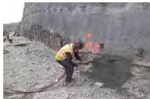
*Contractors are using shotcrete to complete the structural construction phase of a wall below the Food Lion on US 321 in Blowing Rock North Carolina. Image courtesy NCDOT.*
