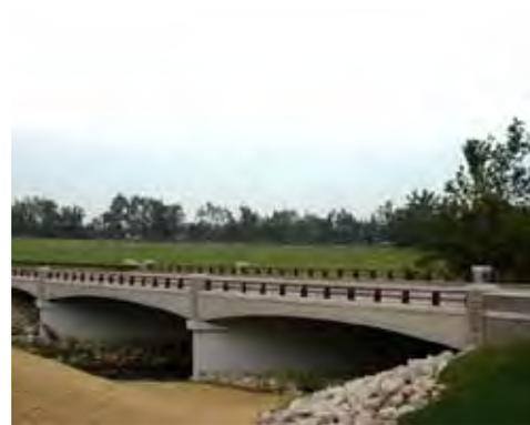
On Paris Pike, which connects Paris, Kentucky, to Lexington, Kentucky, the new bridge over North Elkhorn Creek has a low profile that blends with the landscape. The light gray concrete, stone abutments, simple columns, and open rail are all part of the bridge aesthetics. Image courtesy Wikipedia Commons.
