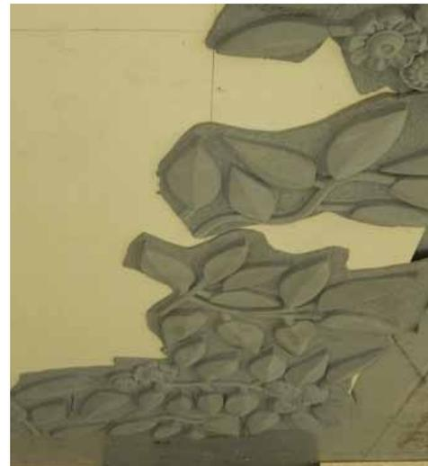
*Grass pattern design by Braaksma Design Inc is one of several design treatments on precast concrete retaining walls and noise abatement walls for Denver's Transportation Expansion Project of the I-25 Corridor; the imagery is based on history, geography and ecology of the Denver region.*
