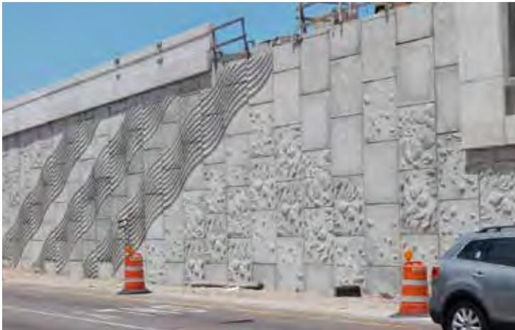
*Wavy diagonal lines and patterns that look like shells and other sea elements are used for a precast concrete retaining wall at the intersection of US 19 and SR 60 in Clearwater, Florida. Image courtesy Creative Design Resolutions.*
