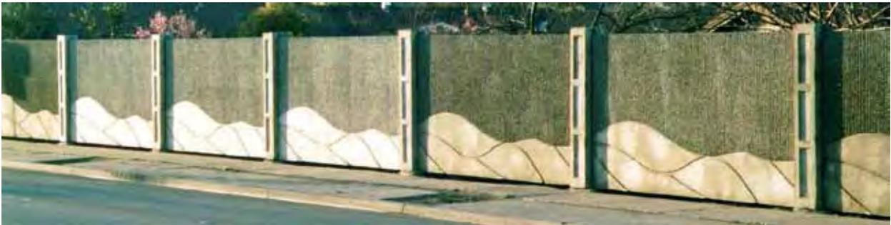
*These precast concrete panels represent a rolling landscape on the bottom and an infinite sky on the top, represented by darker horizontal lines. Image courtesy FHWA.*
