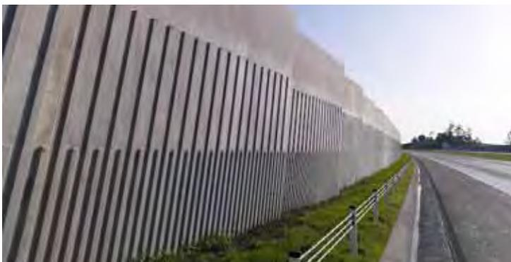
*This noise wall in Bonville, New South Wales, is at a slight angle so that adjacent panels have an offset from the previous panel. An angular pattern is used to decorate the wall. Image courtesy EDAW.*
