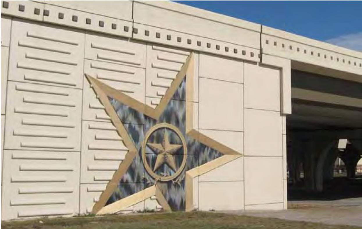
*For this wall in Texas, Texas DOT included the Texas Star as part of the retaining wall that serves as an abutment for this bridge. The wall is made of MSE modules that either have a smooth surface or offsetting horizontal bars to add visual interest. The Star is part of seven different MSE modules. Image courtesy Customrock.*
