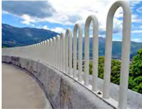
This modern interpretation of rails includes u-shaped arches connected to a metal rail at the top of a stone retaining wall. Image courtesy DepositPhotos.com.
