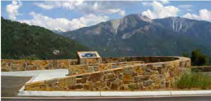
*This scenic overlook is constructed of native stone masonry. Image courtesy FHWA.*
