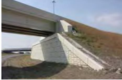
*End bent MSE wall for a bridge over I-75. Image courtesy James Sipes.*
