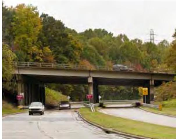
*A steel girder bridge is one of the basic NCDOT bridge standards. Image courtesy FHWA.*
