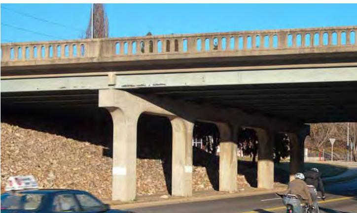
*This bridge abutment has a stone pattern surface to add visual interest by using a finer texture and warmer color. Image courtesy NCDOT.*
