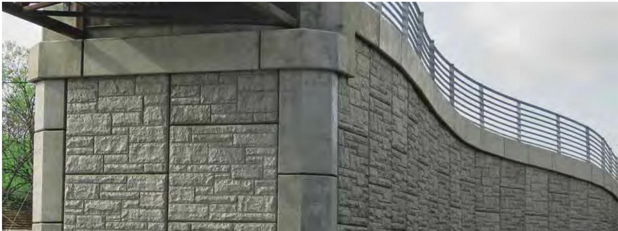
*This bridge abutment is constructed of MSE panels with form lined stone pattern surfaces. Image courtesy James Sipes.*
