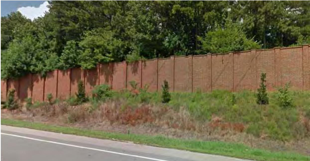
*This brick noise wall is installed along U.S. 540 in Raleigh, North Carolina. The mature vegetation behind the wall and the newer vegetation in front help reduce the visual impact of the wall. Image courtesy James Sipes.*
