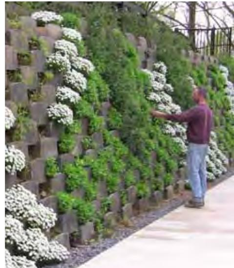
*The use of keystone blocks or other materials that provide openings can be used to develop a green wall. Image courtesy EDAW.*
