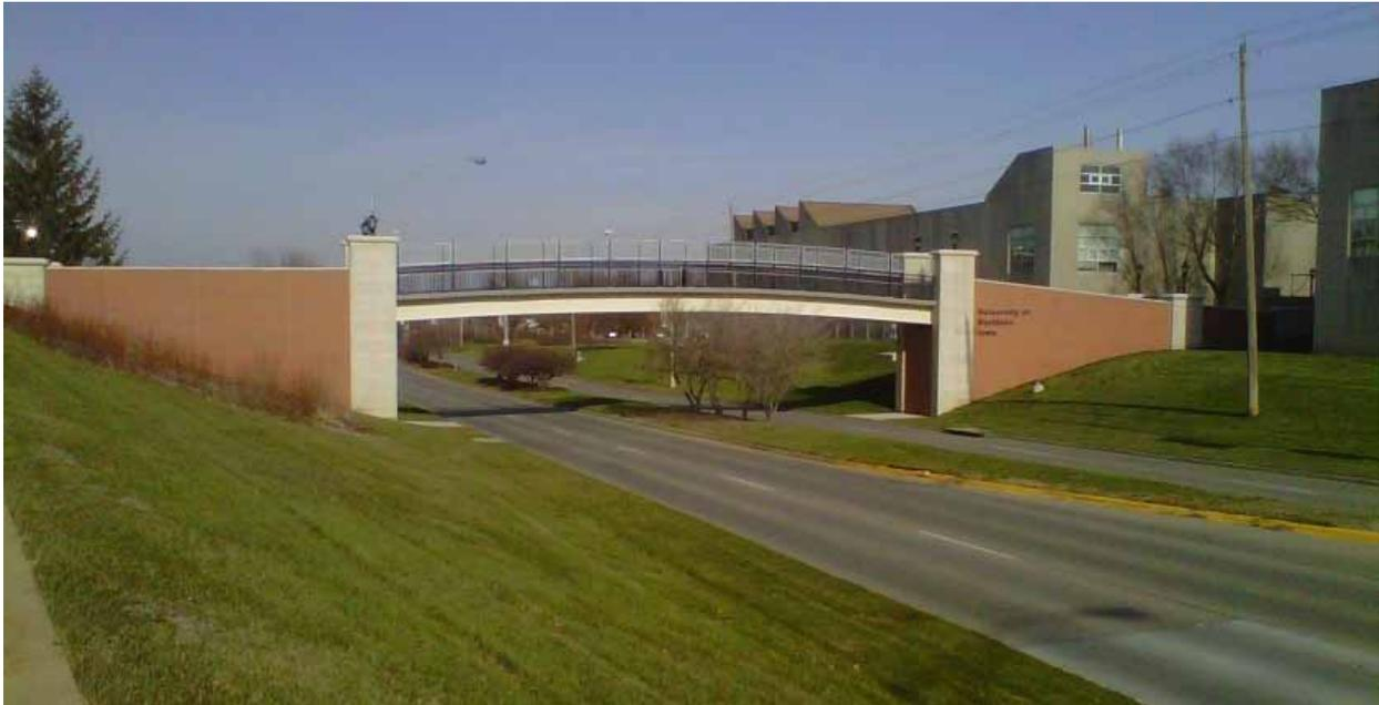
*The Hudson Road Overpass 90' x 11' steel beam pedestrian bridge for the University of Northern Iowa. Aesthetic improvements included brick and limestone treatment, decorative steel railing, galvanized safety railing, handrail and decorative lighting. Image courtesy Snyder Associates.*
