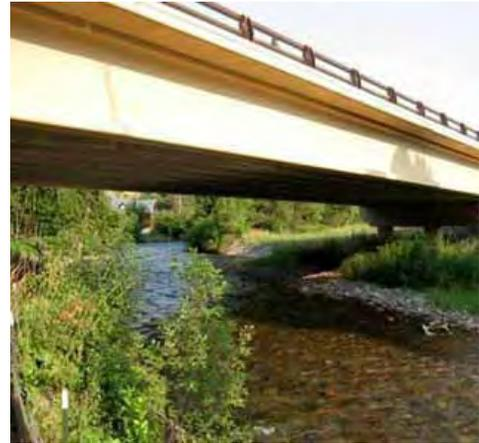
*The Jocko River Bridge along U.S. 93 on the Flathead Indian Reservation in northwest Montana is simple in design so it doesn't distract from the surrounding landscape. It is also designed with sufficient height and span to allow for the continuation of ecosystems and the crossing of wildlife. The incorporation of wildlife considerations makes this bridge a more integrated solution than is normally used. Image courtesy MTDOT.*
