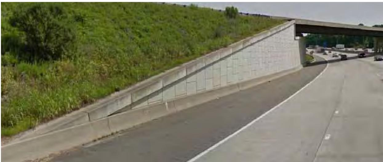
*These retaining walls are used to create bridge abutments that structurally support the bridge over the roadway and stabilize the adjacent slopes. These walls are made of modular MSE panels outlined by concrete caps. A standard jersey barrier is located in front of the wall. Image courtesy James Sipes.*
