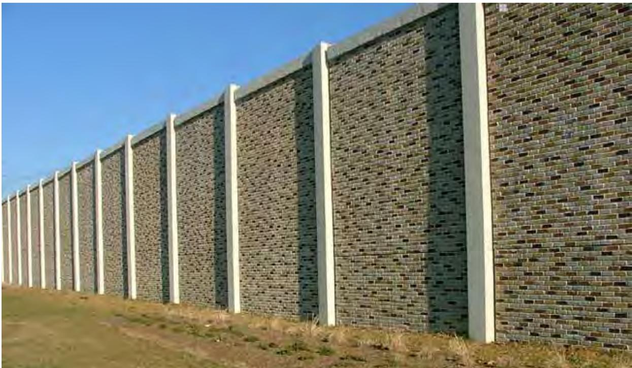
*This wall is constructed of light-colored concrete piers and cap, and precast panels created with used brick form liner. Image courtesy Customrock.*
