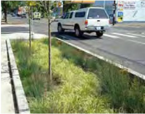
*This bioswale in Seattle, Washington uses a mixture of native grasses to create a visually exciting solution for stormwater runoff. Image courtesy EDAW.*
