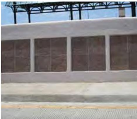
*In Arlington, Texas, precast concrete walls separate pedestrian from vehicular traffic on some of the city's major bridges. The darker panels in the walls provide a greater level of visual detail and is consistent with other details of the bridge. Image courtesy NCDOT.*
