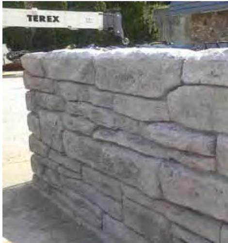
*This is a test panel constructed for a proposed aesthetic wall treatment on US 321 in Blowing Rock, North Carolina. The test panel shows the color, texture, and detail of the front panel and the top of wall treatment. The basic idea behind a test panel is to ensure that the wall, as constructed, is consistent with the design for the wall. Image courtesy NCDOT.*
