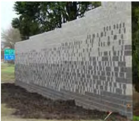
*As part of the Willamette (OR) Passage Bridge, which opened to traffic in August 2013, the project included a new multi-use path, soundwalls, and landscaping. The soundwalls are constructed of light and dark gray concrete masonry units (CMU), with darker CMU blocks on the lower parts of the wall. The changes in color add visual interest without being too distracting. Image courtesy ODOT.*
