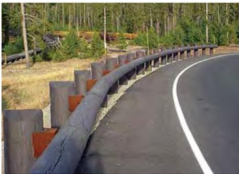
*In Yellowstone National Park, wooden posts and wooden beams connected via steel struts are commonly used as a roadway barrier. Image courtesy FHWA.*
