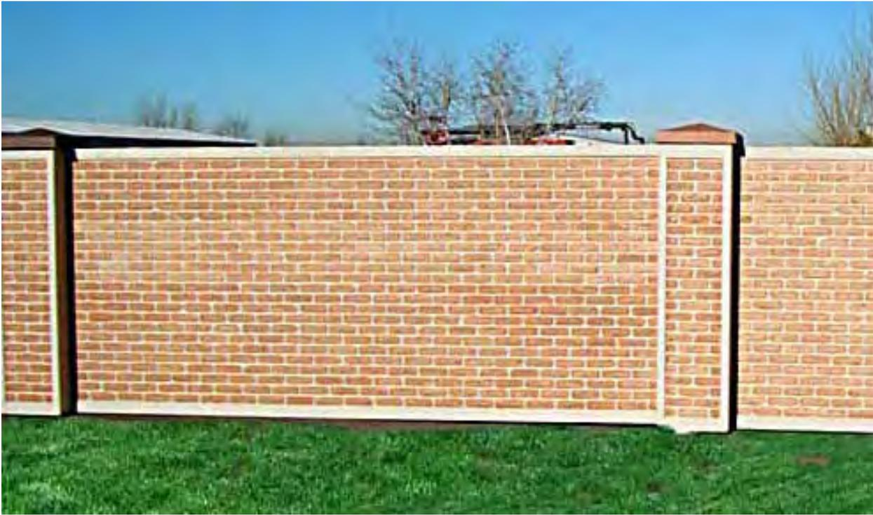
*This is a standard concrete noise wall with form liners used to create the appearance of bricks. The lighter colors on the columns and along the top and bottom of the walls visually fits the 'grout' lines in the panels. Image courtesy FHWA.*
