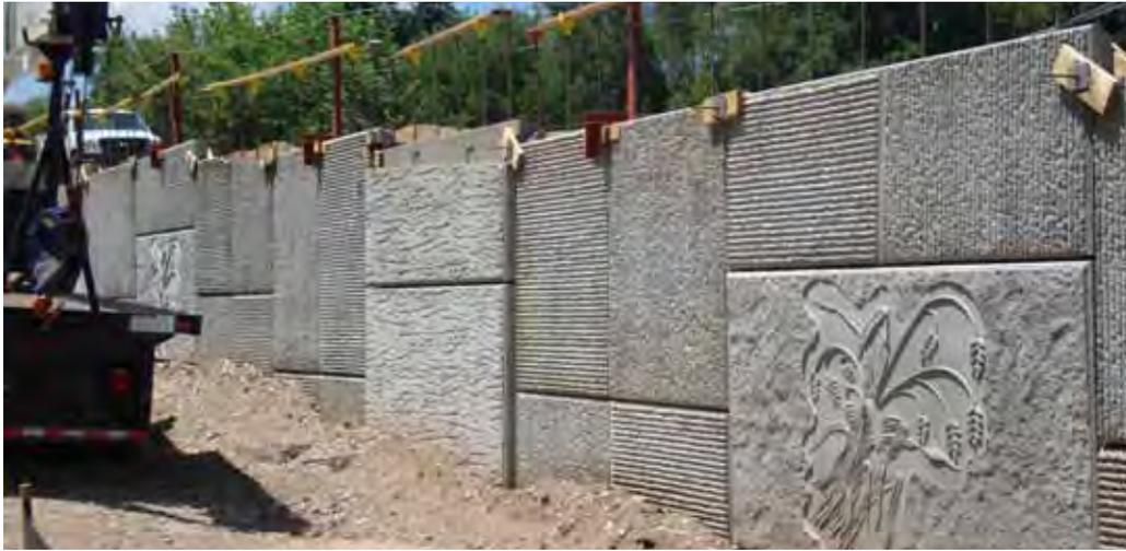
*This image shows the construction of a retaining wall using MSE panels featuring a variety of concrete textures, forms, and colors. The variation in the panels helps add visual interest, but the basic consistency in color and the modular approach to the panels helps provide visual continuity. Image courtesy James Sipes.*
