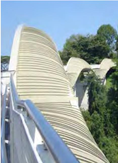
*The Henderson Waves Bridge in Singapore is designed with seven undulating curved steel “ribs” that alternately rise over and under its deck. The unique waveform of the bridge gives it a distinct look. Image courtesy of Wikipedia Commons.*
