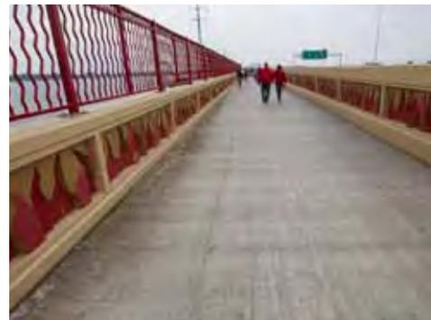
*The Lake Butte des Morts Crossing includes expanded pedestrian crossings as part of bridge structures. For this bridge, the 'fire' them is captured by the graphic elements along both sides of the walkway and the red color and wiggly pattern of the rails. Image courtesy WisDOT.*
