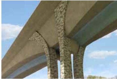
*This is a close-up view of the stone-formed central columns for the Bridge to Nature that are intended to reflect the natural stone found in Vermont. Image courtesy Vermont Transportation.*
