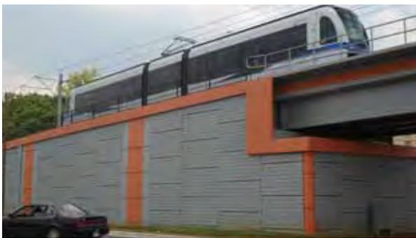
*A reinforced earth MSE precast retaining wall in Charlotte, North Carolina. The red cap and vertical lines creates contrast with the medium gray brick pattern of the precast panels. Image courtesy James Sipes.*
