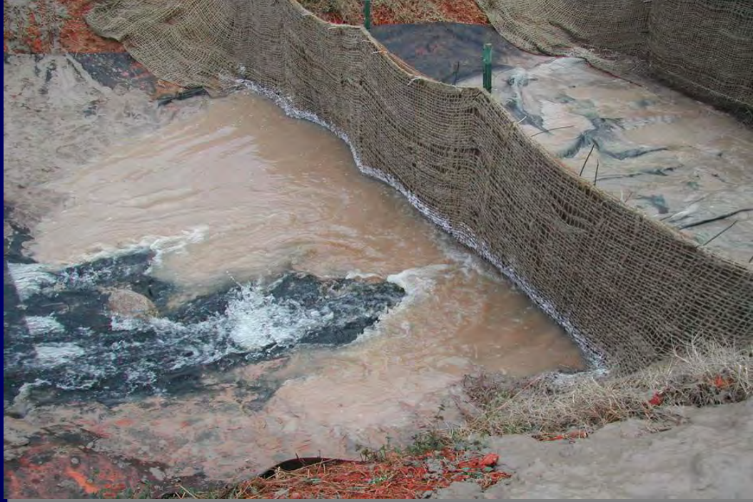
PAM sprinkled on coir baffle in basin (maybe)
