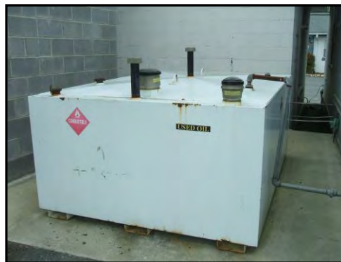
Used oil AST is double-walled
