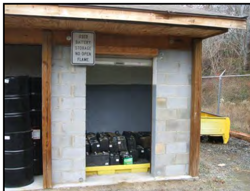
Used batteries stored on spill containment pallet inside building
