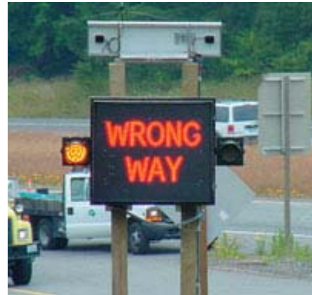
When the sensors determine a vehicle is traveling the wrong way, the message sign illuminates a red "Wrong Way" message
