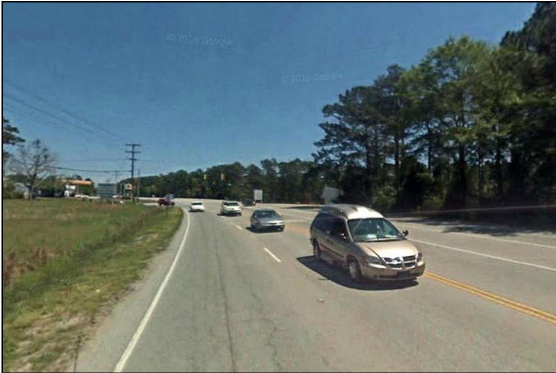
Google Maps (April 2009) – Looking East on NC 24 Approach
