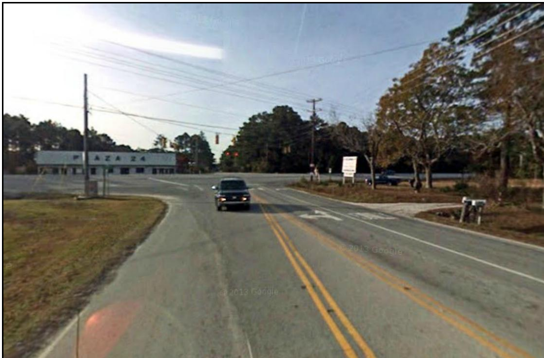
Google Maps (December 2007) – Looking South on SR 1141 Approach
