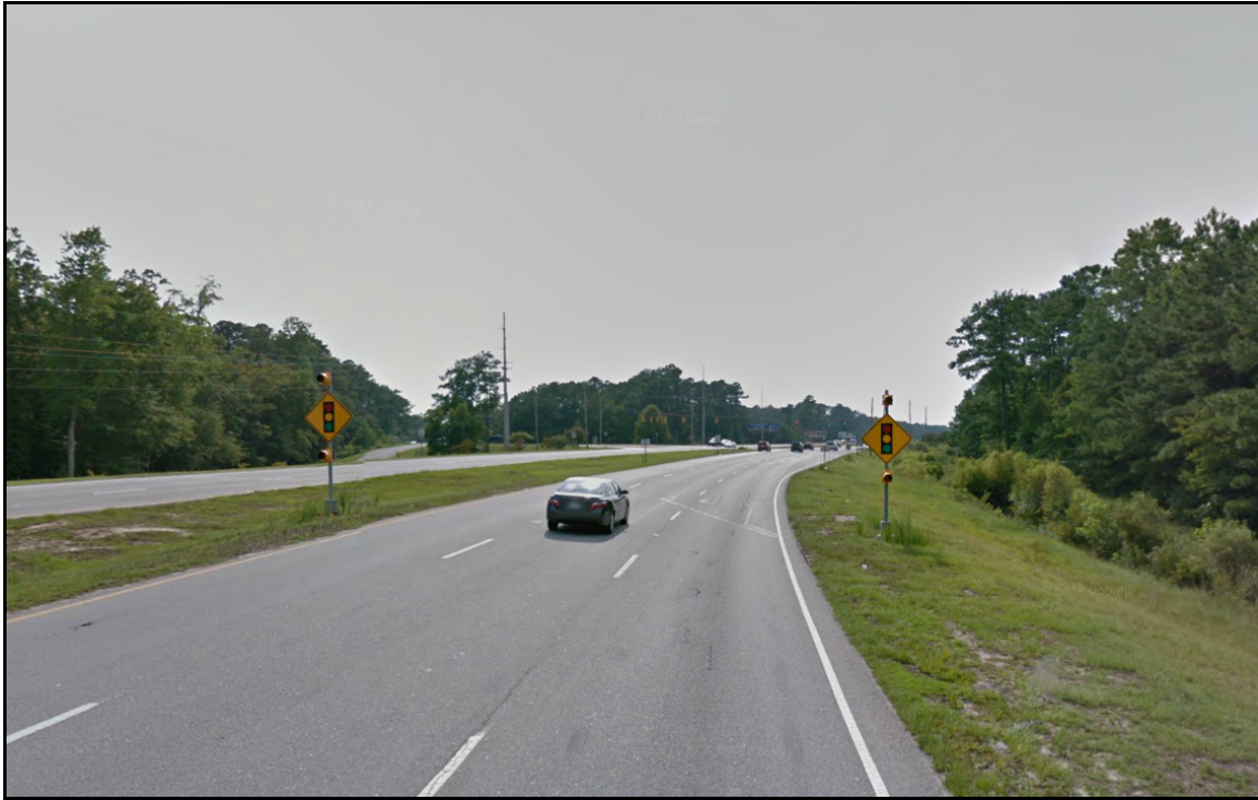
Google Maps (August 2011) – Signal Ahead Signs and Flashers on US 17 Westbound Approach
