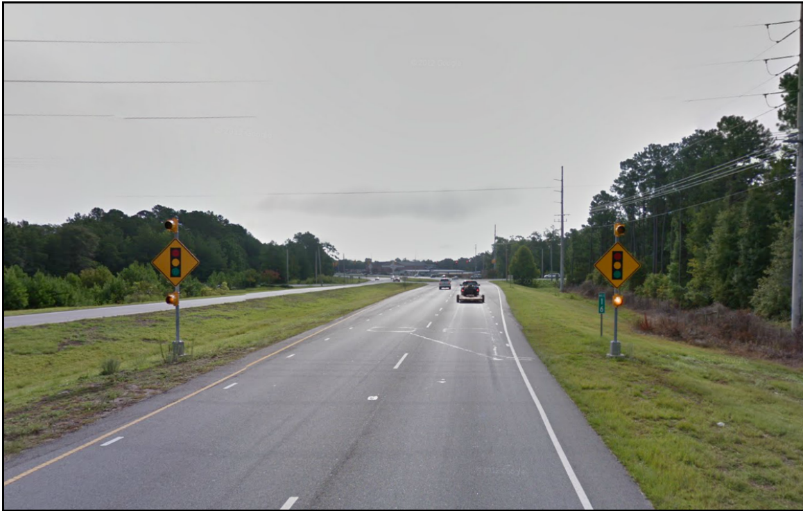
Google Maps (August 2011) – Signal Ahead Signs and Flashers on US 17 Eastbound Approach
