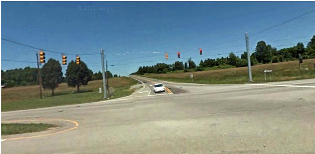
Google Maps (May 2009) – Looking Northeast at SR 1601
