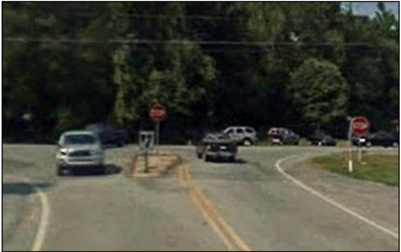
Google Maps (May 2008) – Looking North from SR 1952 (White Cross Rd) Approach
