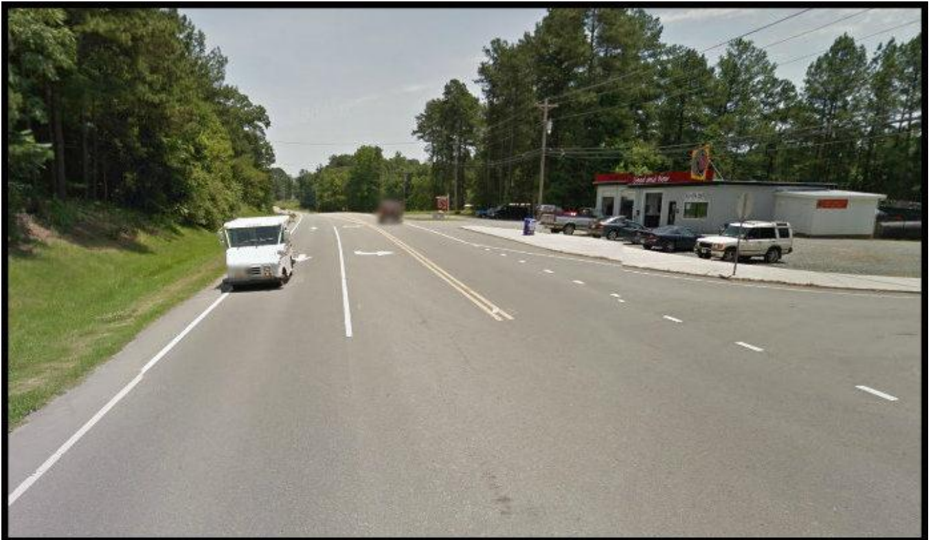
Google Maps (May 2012) – Looking East from NC 54 Approach
