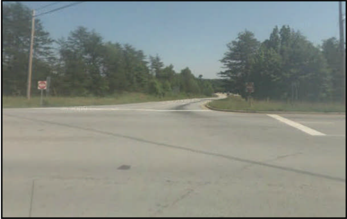
Google Maps (June 2009) – Looking South on US 21 Approach
