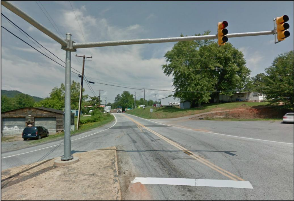
Google Maps (May 2012) – Looking Northwest on NC 9 Approach
