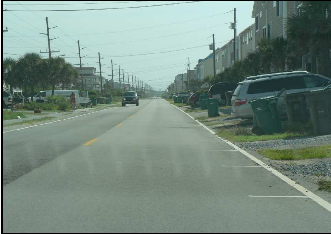
Installed Countermeasure Site 4 / Treatment 2 – South Shore Drive Combined Area Pavement Markings on Both Sides of Roadway
