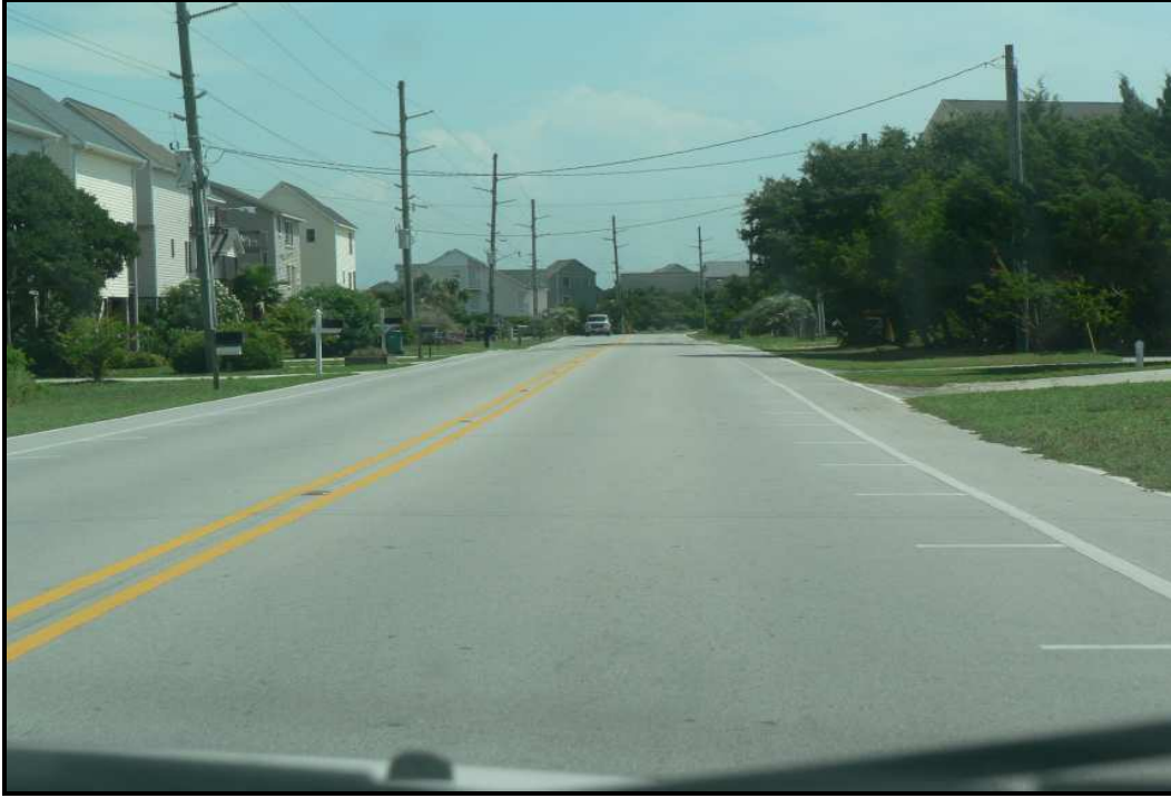
Installed Countermeasure Site 3 / Treatment 1 (South Topsail Drive) Combined Area Pavement Markings on Both Sides of Roadway
