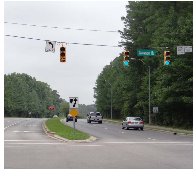
Figure 4D-7. Typical Position and Arrangements of Separate Signal Faces with Flashing Yellow Arrow for Permissive Only Mode Left Turns
