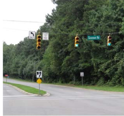
Figure 4D-12. Typical Position and Arrangements of Separate Signal Faces with Flashing Yellow Arrow for Protected/Permissive Mode and Protected Only Mode Left Turns
