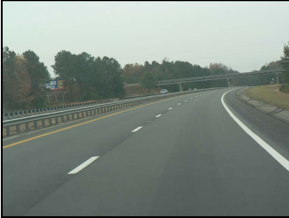
Traveling South on I-95 at SR 1202 Bridge
