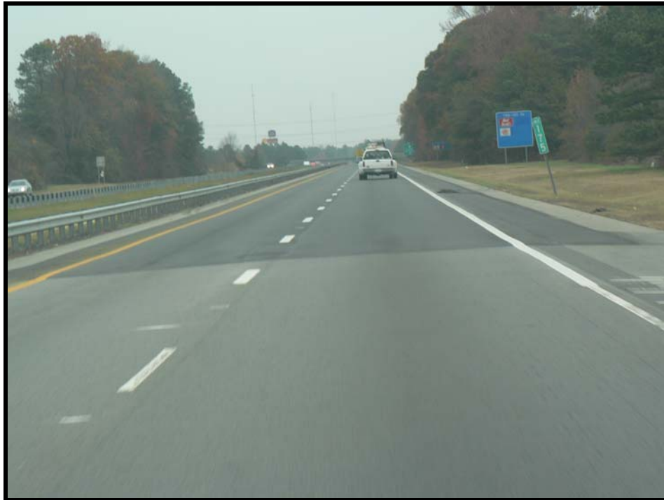
Beginning of Resurfacing Project (Traveling NB)
