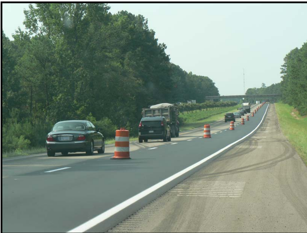
Dump Truck led platoons – assisted in regulating speeds
