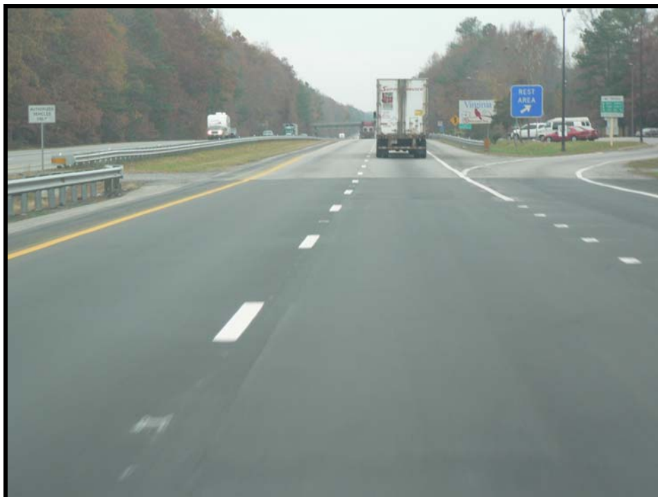
End of Resurfacing Project at Virginia Border (Traveling NB)
