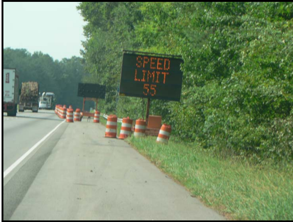
Speed Reduction CMS at beginning of Workzone
