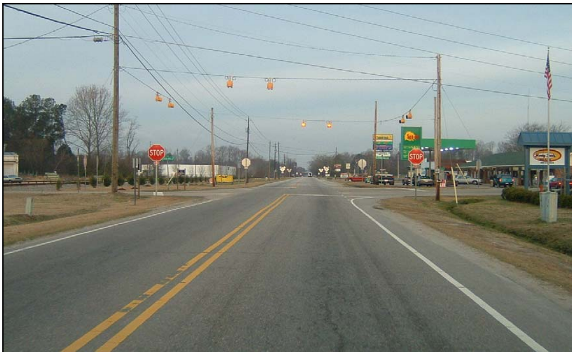
Looking West on SR 1006 (Clinton Rd)
