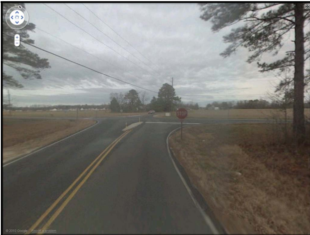
Looking north on SR 1127 (Frog Level Rd)
