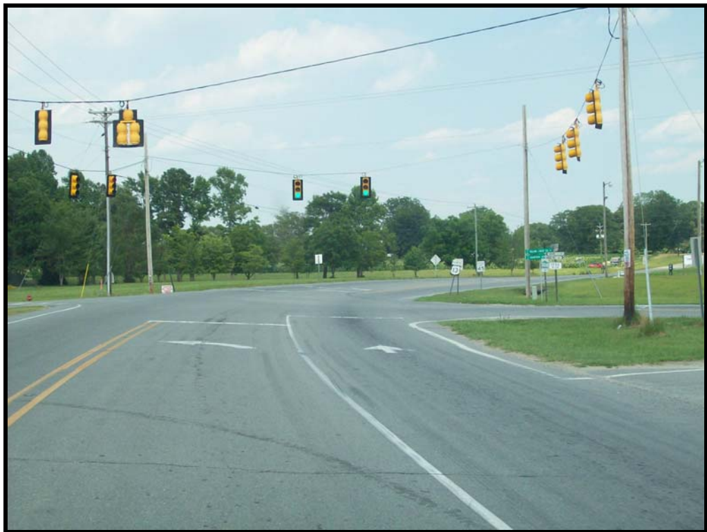
Traveling East on US 13 (Notice Channelization Ramp to right)
