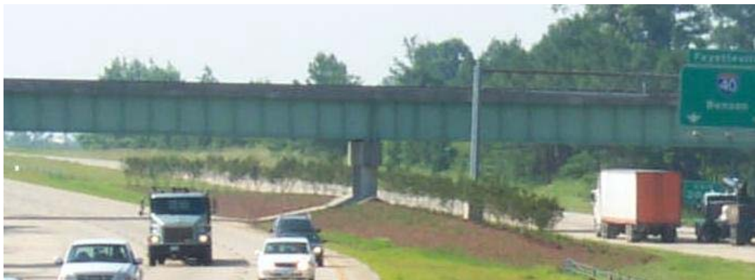
Figure 1. Typical Median Berm
