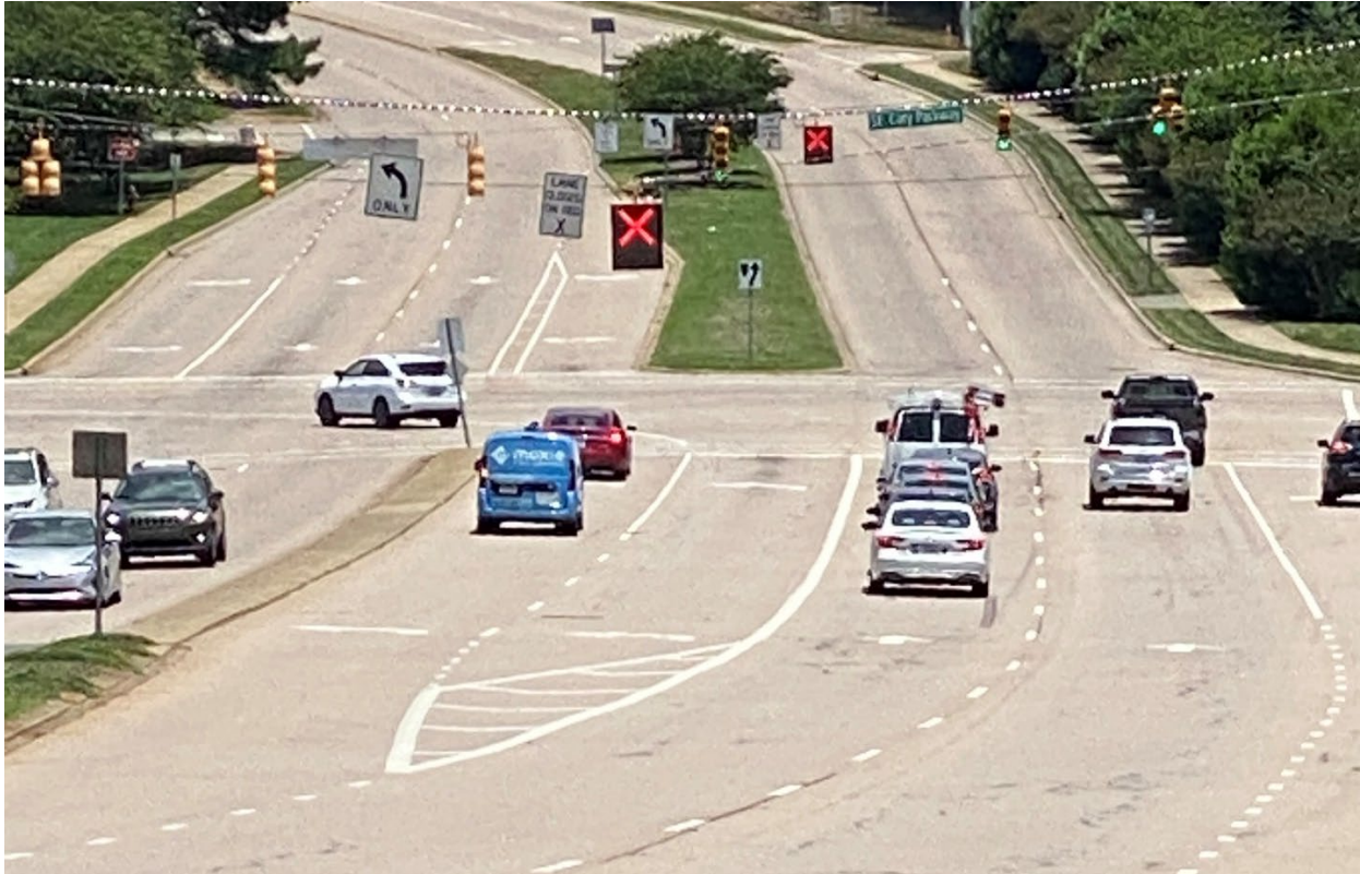
Figure 23. Main traffic control devices for the DLTi.
