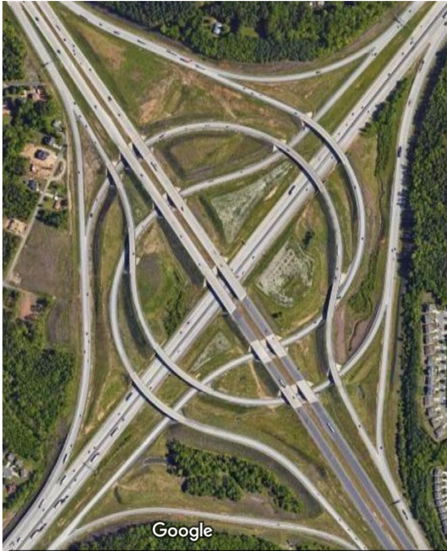
Figure 30. Turbine interchange at I-85 and I-485 in Charlotte.
