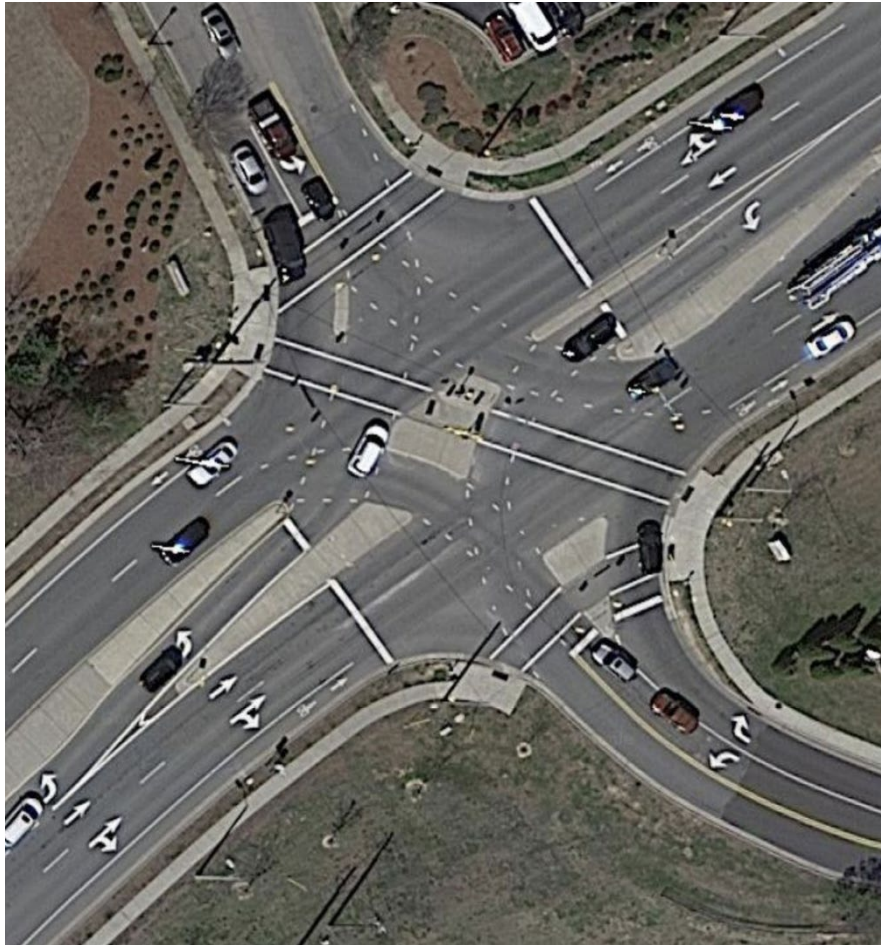
Figure 18. Thru-cut intersection at South Main Street and Village Walk Drive in Holly Springs, NC.
