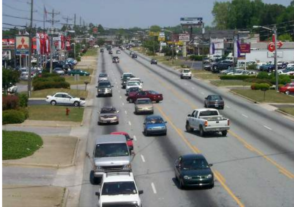
Figure 4. Segment of Five-Lane Road with TWLTL
