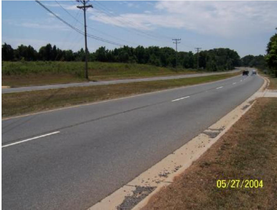
Figure 30. Westbound NC 24-27 (0.7-mile rural corridor)
