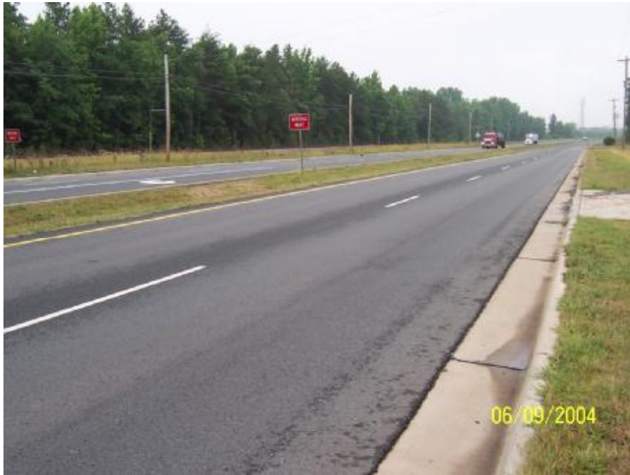
Figure 29. Westbound NC 24-27 (1.9-mile rural corridor)
