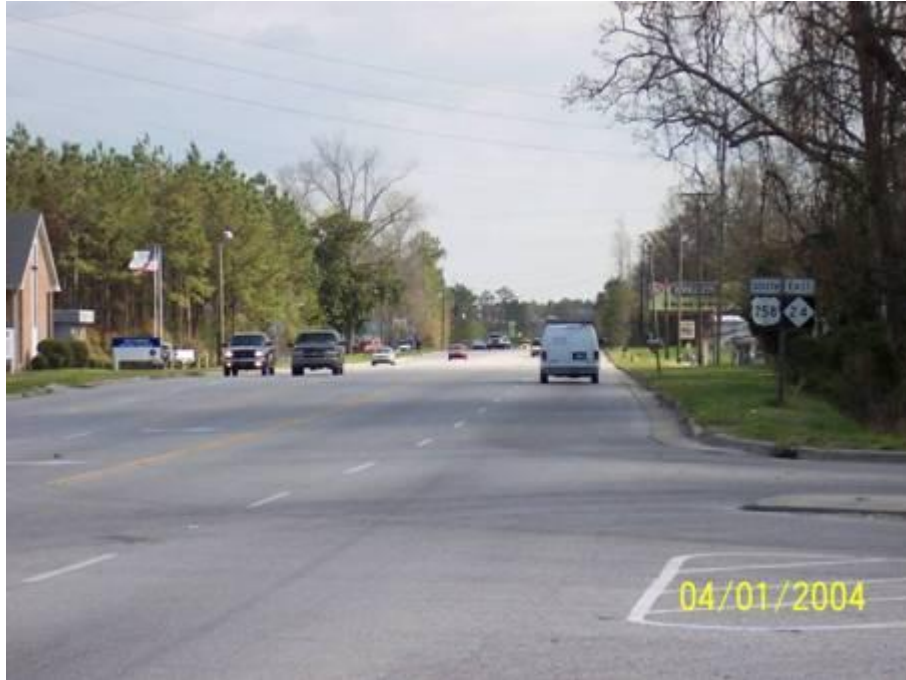
Figure 40. A site with a 55 mph speed limit and TWLTL median (US-258 and NC-24 in Onslow County)
