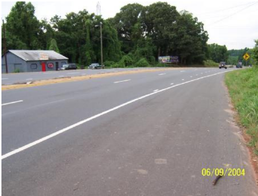
Figure 26. Westbound US-29 in Division 10
