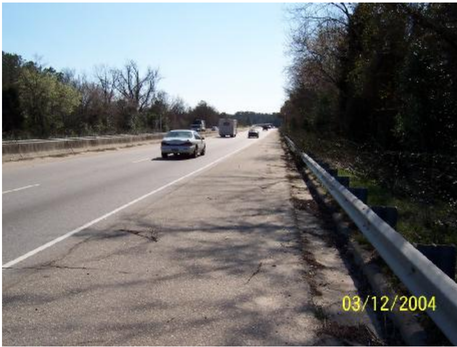
Figure 19. Southbound US-401 Business
