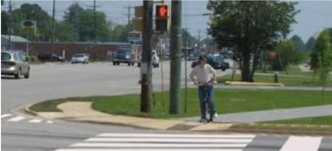
*Figure 4 Sidewalk, ramps, and detectable warnings at this corner serve as an ADA compliant path.*
