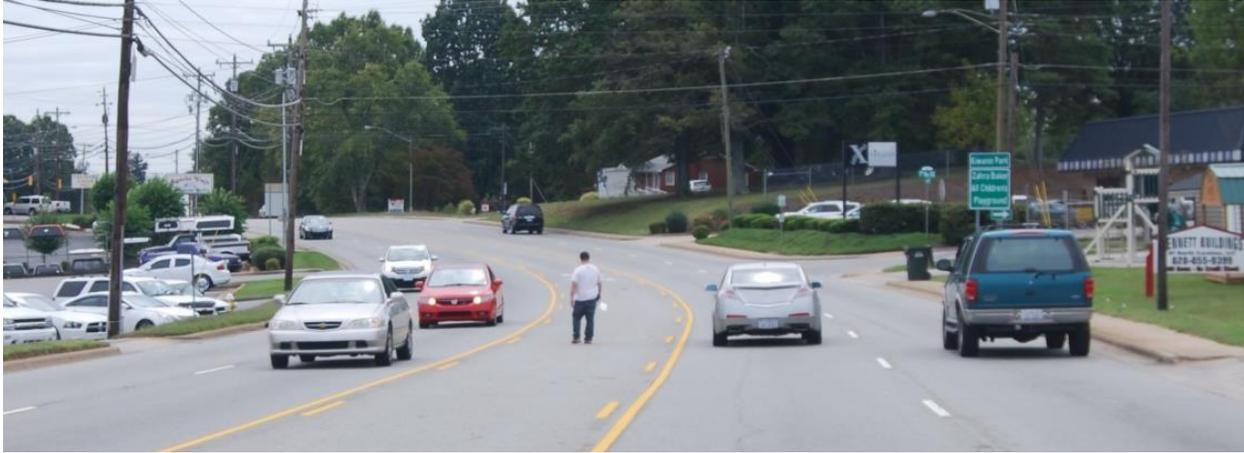
Figure 11 On roads with 4 or more lanes without a raised median, if the posted or operating speed is 35 mph or more, marking a crosswalk alone is not recommended. Even if vehicle speeds are 30 mph or less, if the traffic volume is greater than 9,000 vpd, marking a crosswalk alone may increase the risk of a pedestrian crash. Instead, additional/alternative treatments should be considered.
