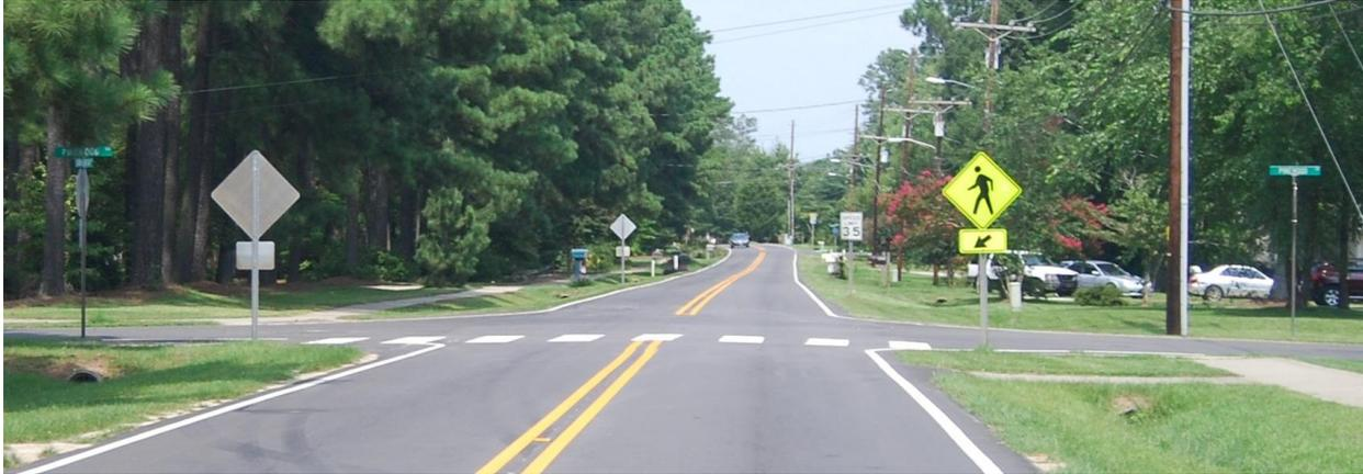
Figure 10 At an unsignalized intersection, if the posted or operating speed of a two-lane road is greater than or equal to 40 mph, marking a crosswalk alone is not recommended as it may increase the risk of a pedestrian crash.
