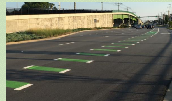
GREEN-COLORED PAVEMENT FOR BICYCLE FACILITIES
