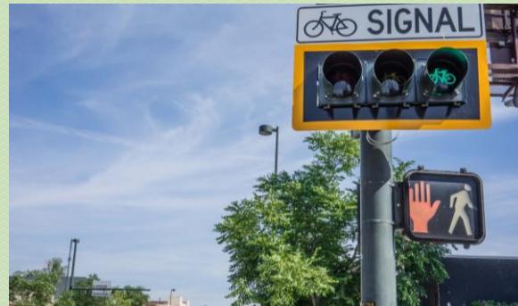
SIGNAL IMPROVEMENTS FOR BICYCLES (INCLUDING SIGNAL TIMING, BIKE SIGNALS)
