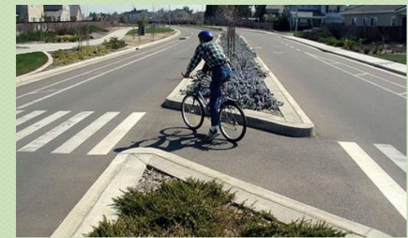
MEDIAN AND CROSSING TREATMENTS FOR BICYCLES
