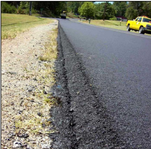
SR 1611 in Burke County: Resurfacing With Safety Edge
