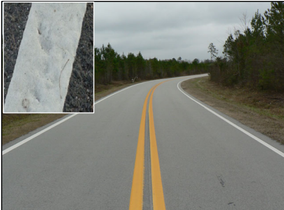
6” Wide Markings with Standard Beads SR 1004/ Island Creek Rd in Jones County
