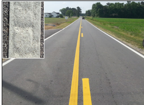
6” Wide Markings with Highly Reflective Elements SR 1306/Beautancus Rd in Duplin County
