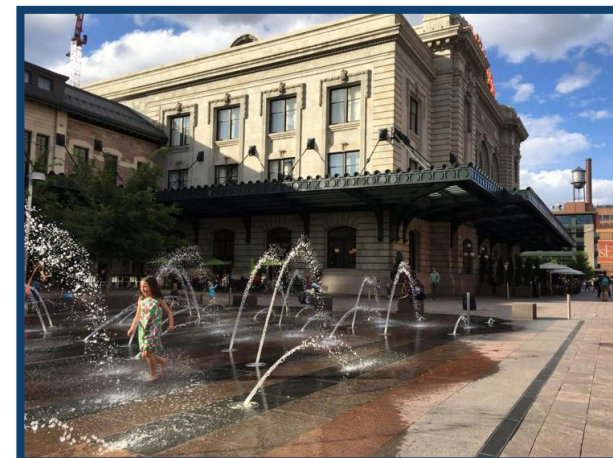
Denver Union Station at Wynkoop Street
