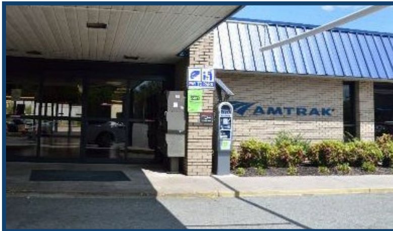
Main entrance to Staples Mill
