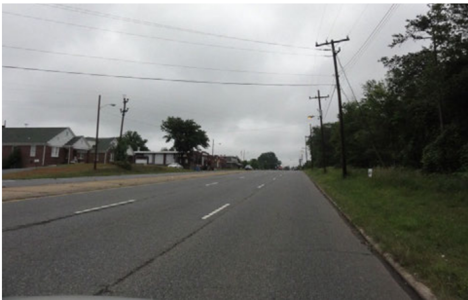
Figure 3-4. Highway 74 current conditions
