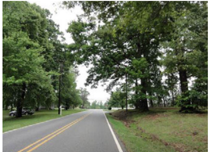
Narrow roadways and lanes
