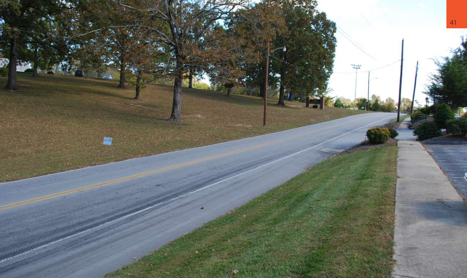
GROVE STREET — EXISTING
