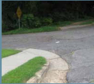
No crosswalks, no curb cut on one side:
