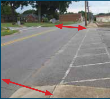
Crosswalks that parallel major streets but none that cross them:
