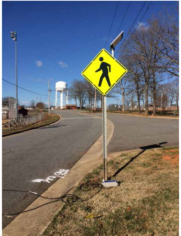
Other recent intersection improvements include the installation of flashing pedestrian signs along East 22nd Street near Northside/Broyhill Park.
