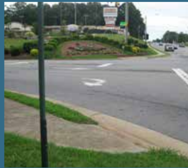
Pedestrian signal and sidewalks, but no crosswalk:
