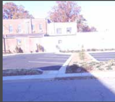
Poor connectivity through parking lots to access business entrances
