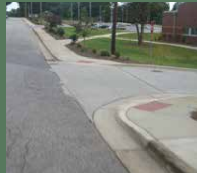
Great new sidewalks at South Newton Elementary. (However, there are no crosswalks or sidewalks on surrounding roads.):
