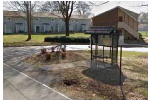
Bus shelter at a Greenways Transit stop on East 1st Street
