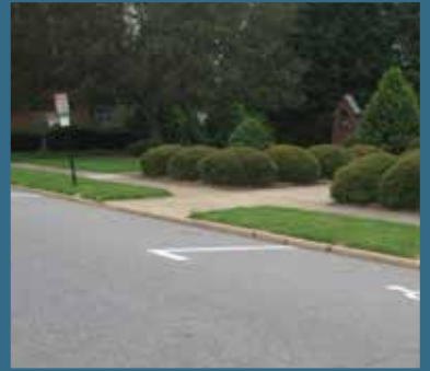
Handicap parking without ramp access:
