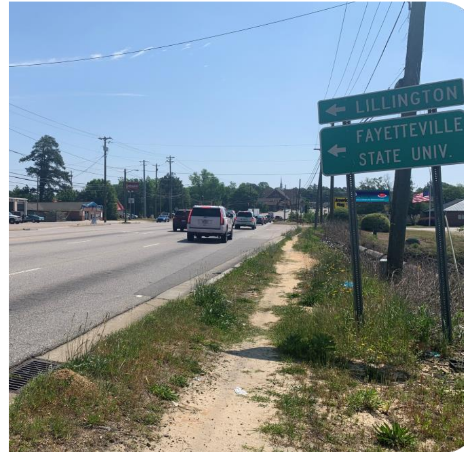
Example of worn path along roadway – Fayetteville, NC
