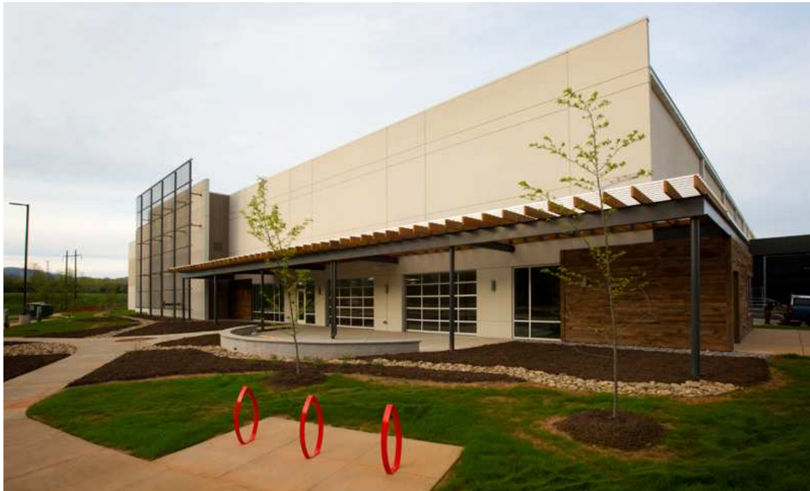
Figure 3.36 New Belgium Brewing Company Distribution Center Asheville
