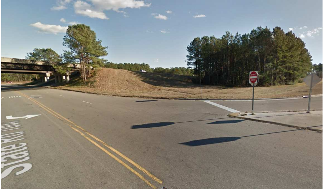
Figure 3.23 I-40 at NC 1002 Southbound Off-Ramp Looking East on NC 1002
