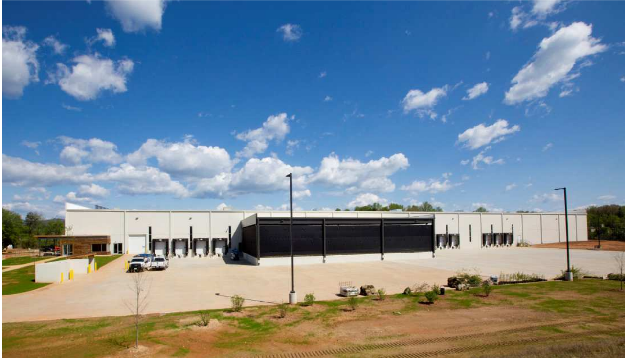
Figure 3.37 New Belgium Brewing Company Distribution Center Loading Area
