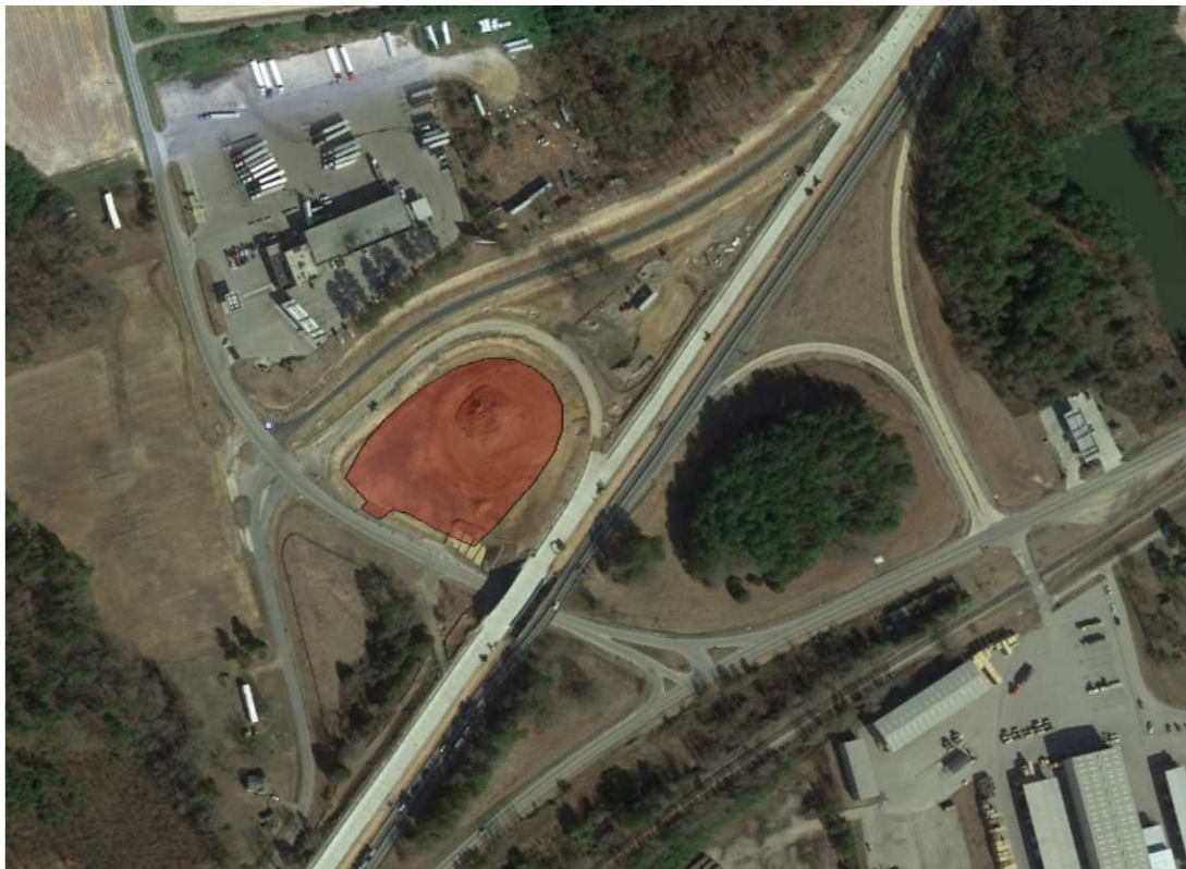
Figure 3.31 I-85 at U.S. 1/Flemingtown Road Vance Co.
