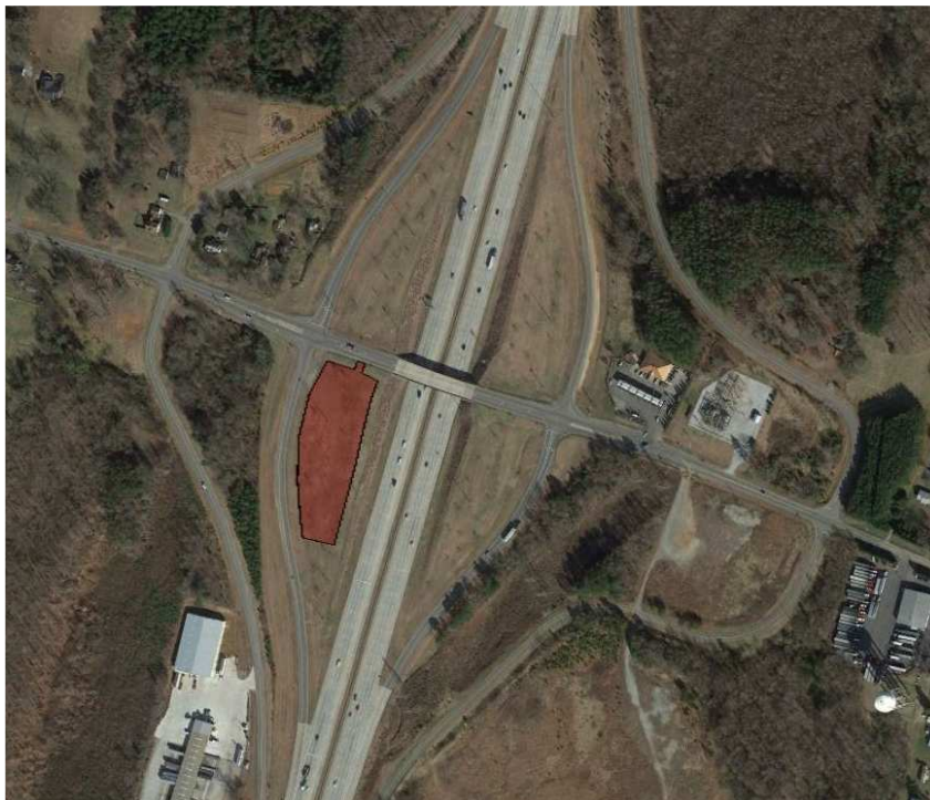
Figure C.32 I-85 at SR 2120 Long Ferry Rd, Rowan County
