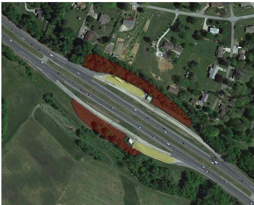
Figure C.7 I-26 at Weigh Station Henderson County
