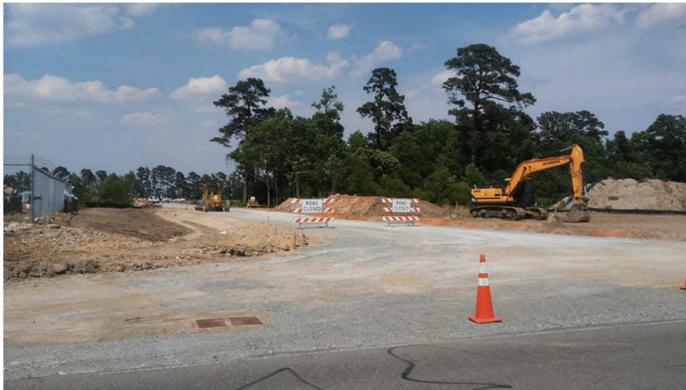
Figure 3.34 Construction of New Road from NC 55 to Mt. Olive Pickle Company
