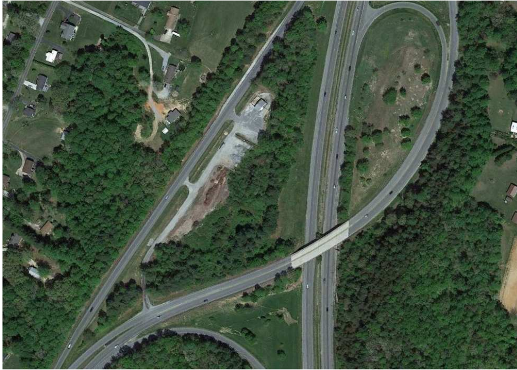
Figure C.8 DOT Storage Yard Henderson County
